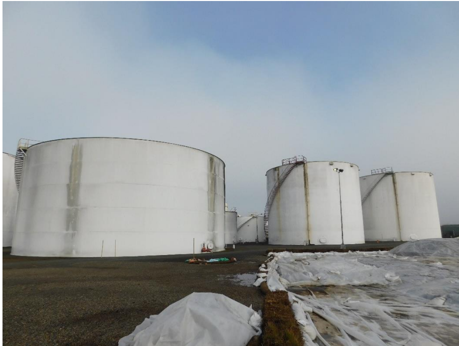
Picture 1. Typical view of tank farm.
