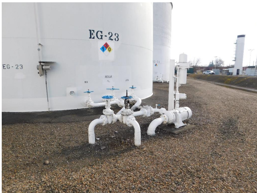
Picture 4. Typical view of buried piping.
