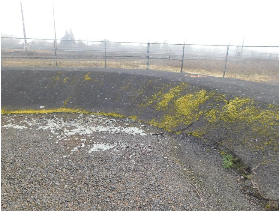
Picture 6. Typical view of gravel berm containment.
