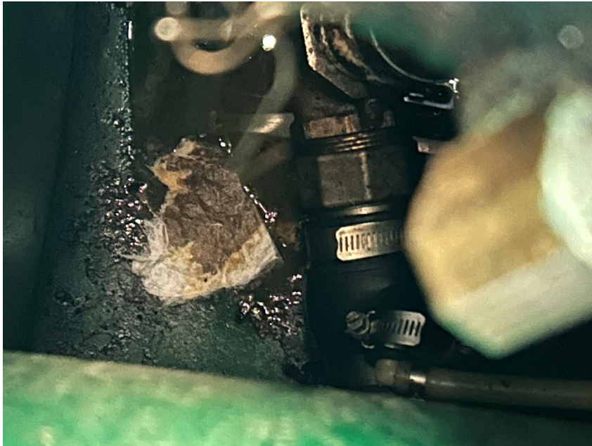
19: Confirmed product in west satellite diesel UDC
