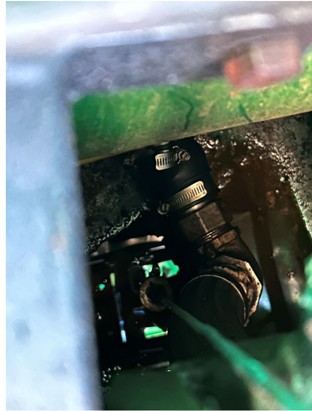
18: West satellite diesel UDC with product present
