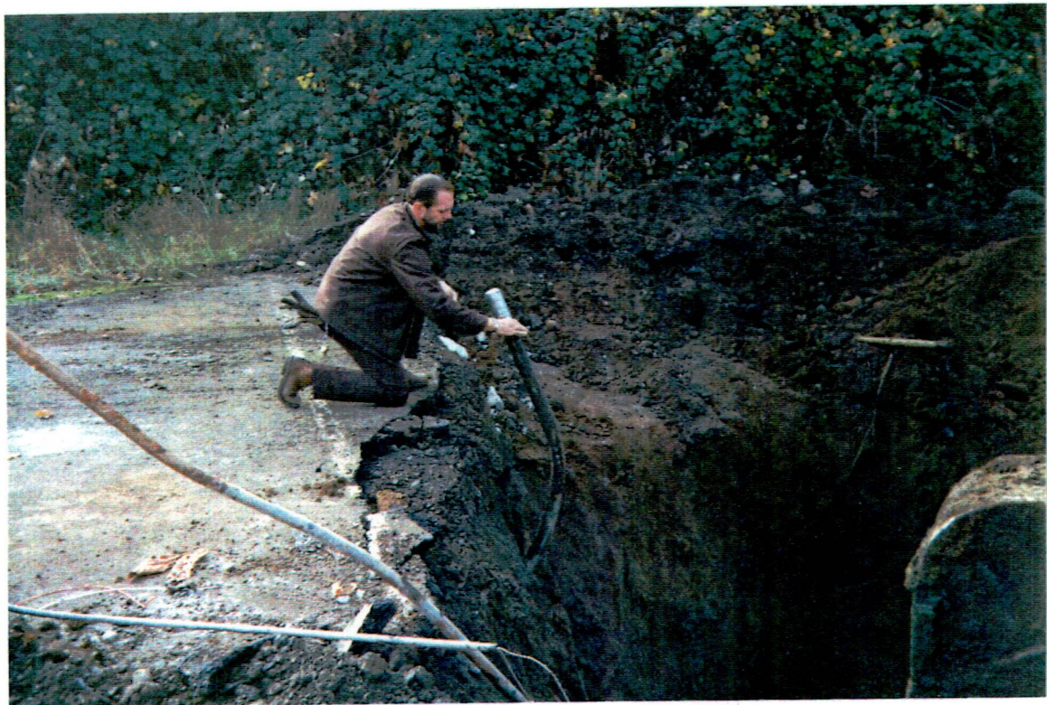
Photograph # 6: Fuel line being sealed by Mr. Norm Davis.
