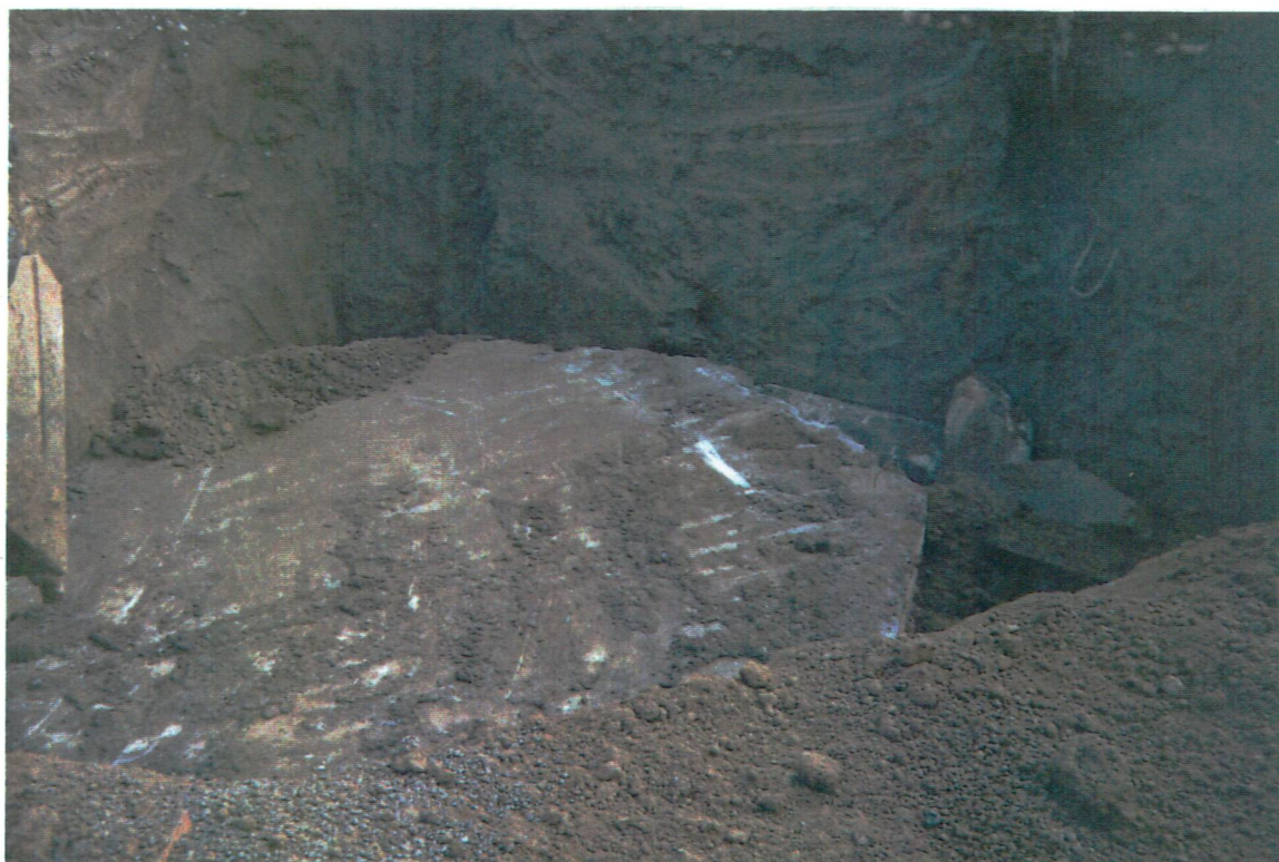
Photograph # 4: View to the east of excavation pit. Note fuel line to the right.
