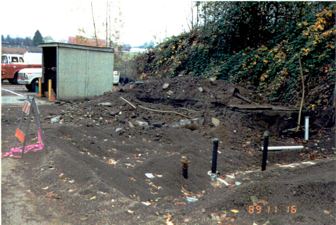
Photograph # 1: View to the east of project site prior to excavation. Note fuel pump shed.
