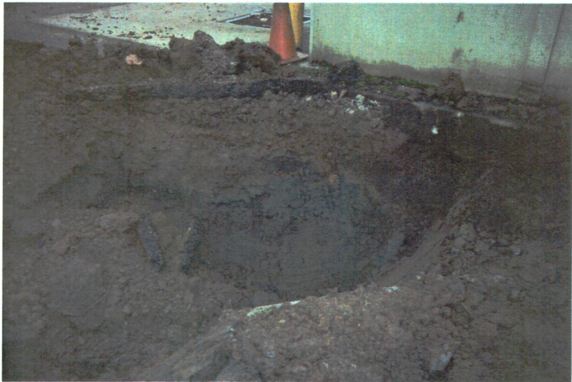
Photograph # 2: Contaminated soil in northeast corner of pit adjacent to pump shed.
