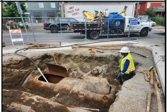
Photo #4: Decommissioning and Cleaning
