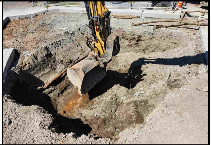
Photo #2: Initial Excavation
