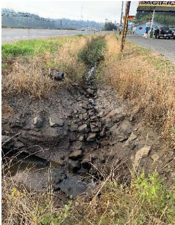
Photo #1 8/30/22 8:29 am: North end of drainage ditch with no observed outflow north of telephone pole 1.5 hours prior to low tide.
