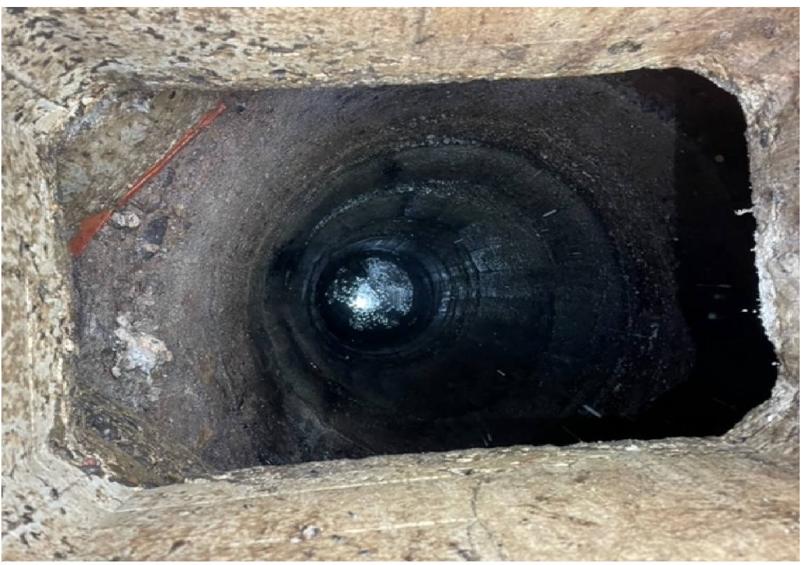
VIEW OF THE CONTENTS OF THE REDLAND STORE'S FORMER UIC FOLLOWING PUMPING ACTIVITIES.
