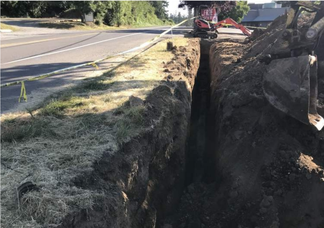
NORTHERLY VIEW OF THE DRAIN PIPE TRENCH, WHERE THE OWNER RE-ROUTED THE NEW LINE USING WATERTIGHT, GASKETED DUAL-WALL PIPING.
