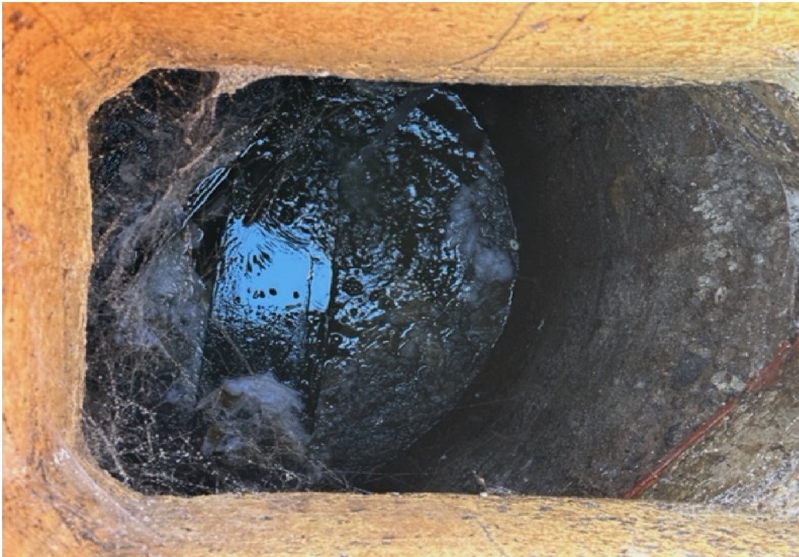
VIEW OF THE CONTENTS OF THE REDLAND STORE'S FORMER UIC PRIOR TO PUMPING ACTIVITIES.
