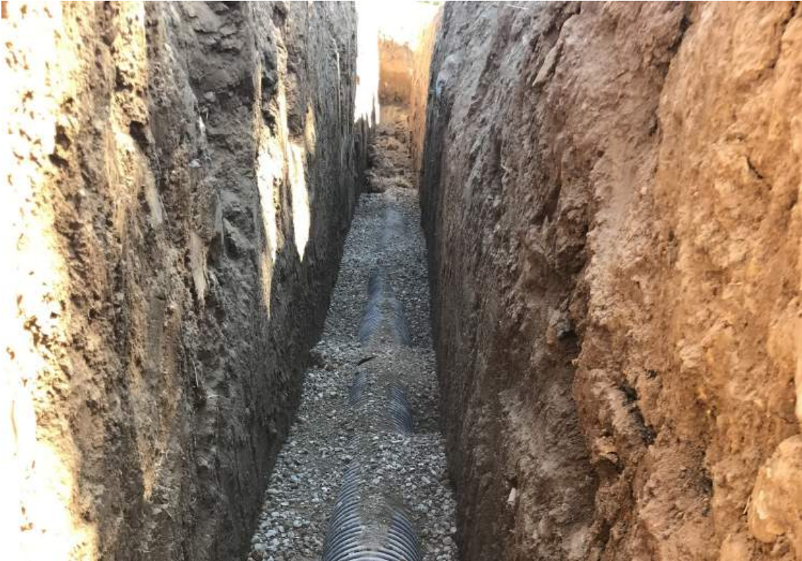
NORTHERLY VIEW OF THE DRAIN PIPE, WHERE THE OWNER RE-ROUTED THE LINE USING WATERTIGHT, GASKETED DUAL-WALL PIPING.
