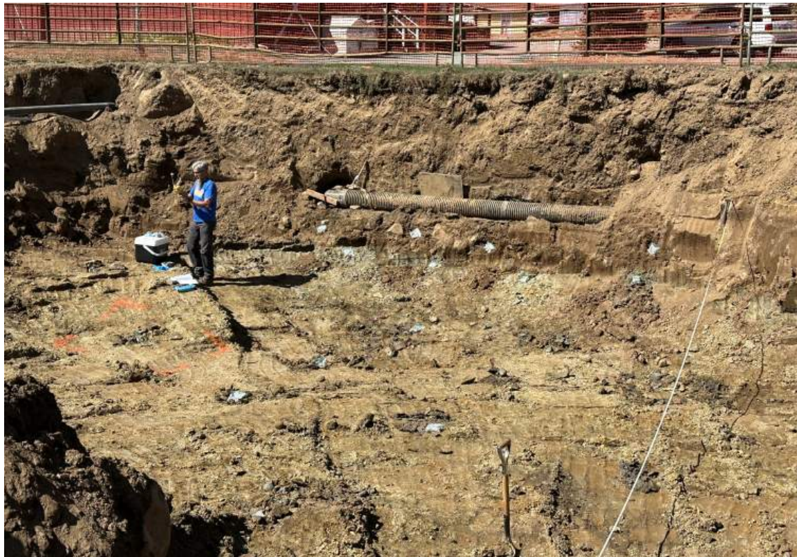
FIELD SCREENING PERFORMED DURING REMEDIAL EXCAVATION ACTIVITIES. PHOTOGRAPH TAKEN FACING WEST.
