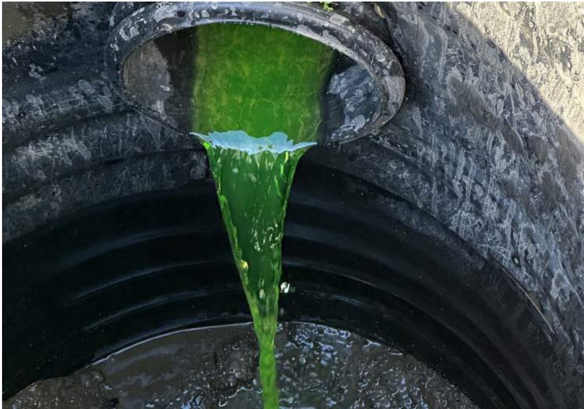
VIEW OF THE GREEN DYE DISCHARGING INTO THE ON-SITE CATCH BASIN FOLLOWING INSERTION INTO THE REDLAND STORE TOILET.
