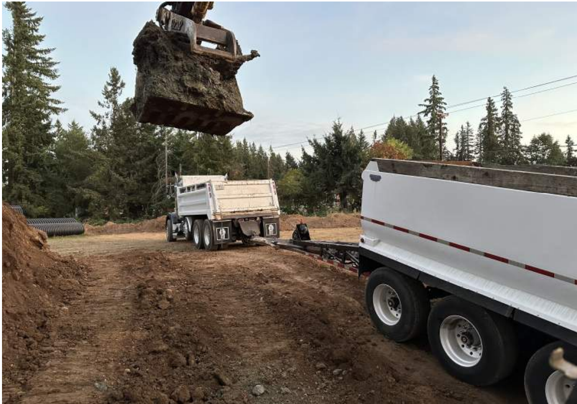
VIEW OF IMPACTED SOIL DISPOSAL DURING REMEDIAL EXCAVATION. IMPACTED SOIL WAS SENT TO THE HILLSBORO LANDFILL. PHOTOGRAPH TAKEN FACING EAST.
