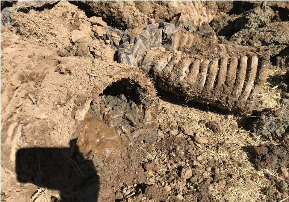
VIEW OF AN EXCAVATED SEGMENT OF DRAIN PIPE THAT WAS REMOVED AFTER THE LINE WAS RE-ROUTED.
