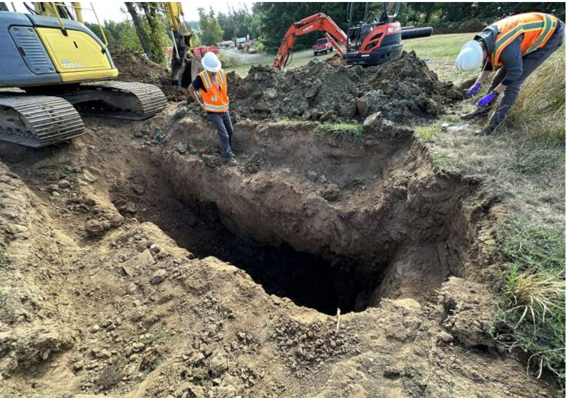
VIEW OF THE ONSITE TEST PIT "TP-1" DURING EXPLORATION. PHOTOGRAPH TAKEN FACING NORTHEAST.
