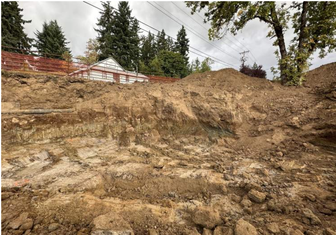
VIEW OF THE FINAL NORTHERN REMEDIAL EXCAVATION LIMITS. PHOTOGRAPH TAKEN FACING NORTH-NORTHWEST.
