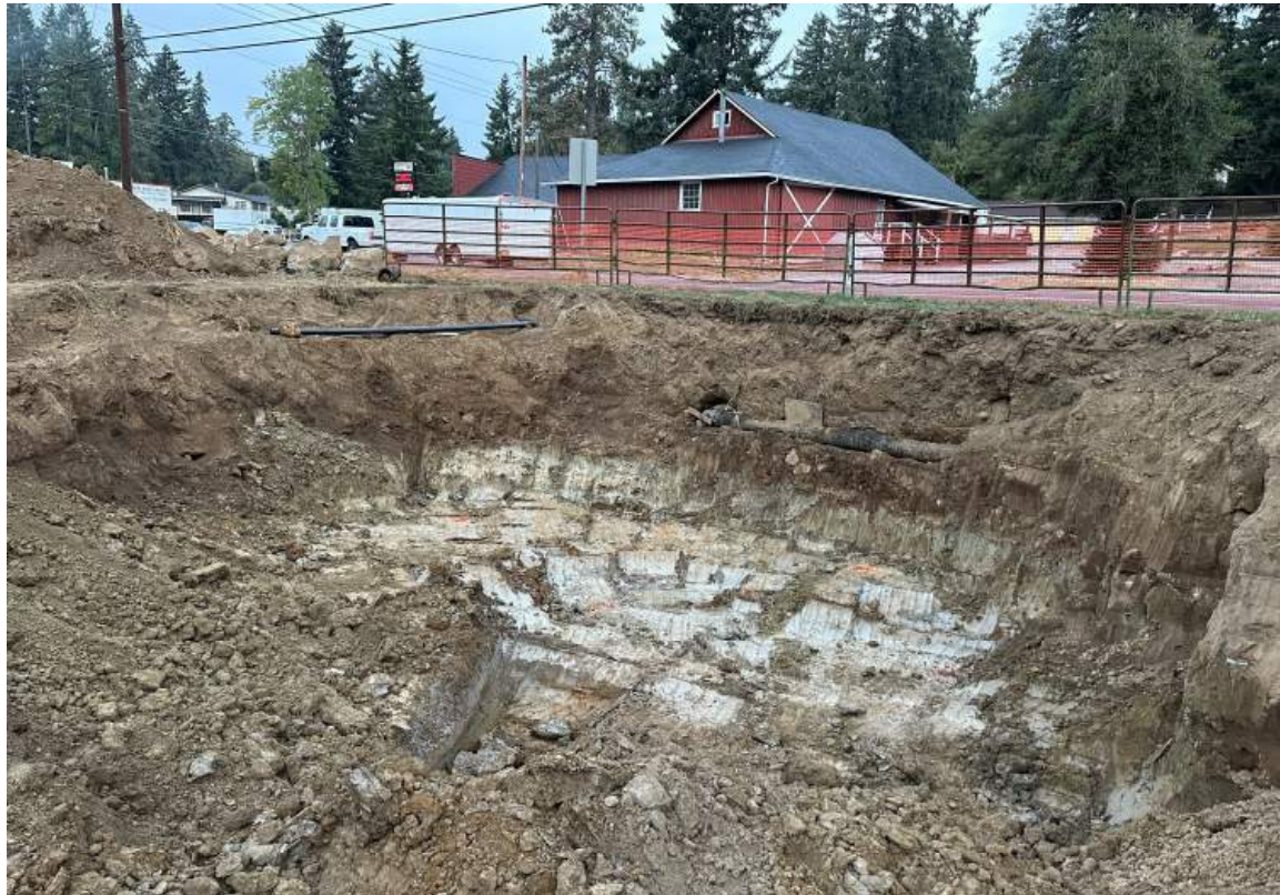
VIEW OF FINAL REMEDIAL EXCAVATION LIMITS AT THE SUBJECT PROPERTY. PHOTOGRAPH TAKEN FACING WEST.
