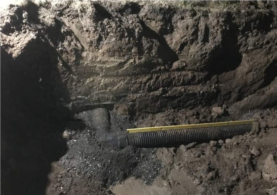
VIEW OF THE DRAIN PIPE, WHERE THE OWNER RE-ROUTED THE LINE USING WATERTIGHT, GASKETED DUAL-WALL PIPING.
