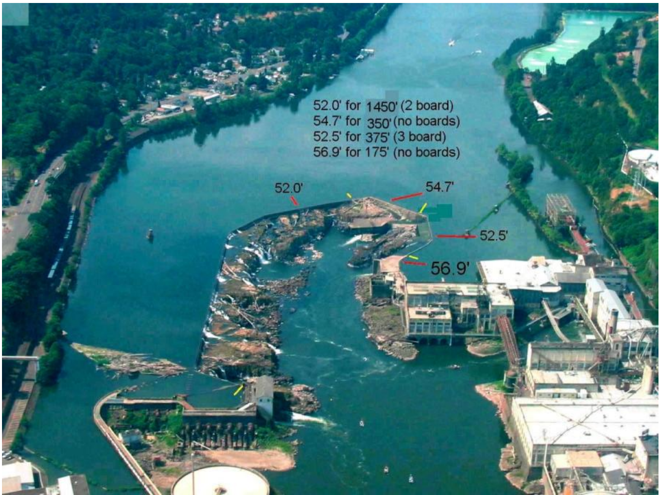
Figure 254. Aerial view of Willamette Falls and dam structures (compliments of PGE)
