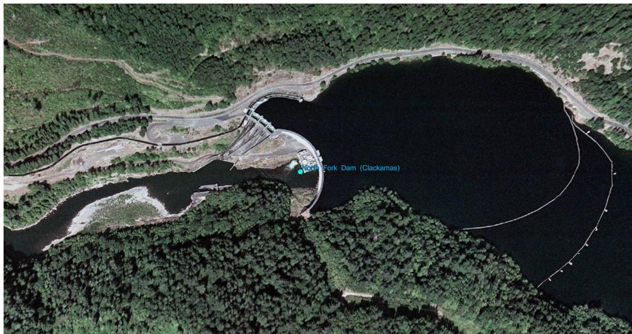
Figure 5-7. PGE's North Fork Dam and Reservoir on the Clackamas River
