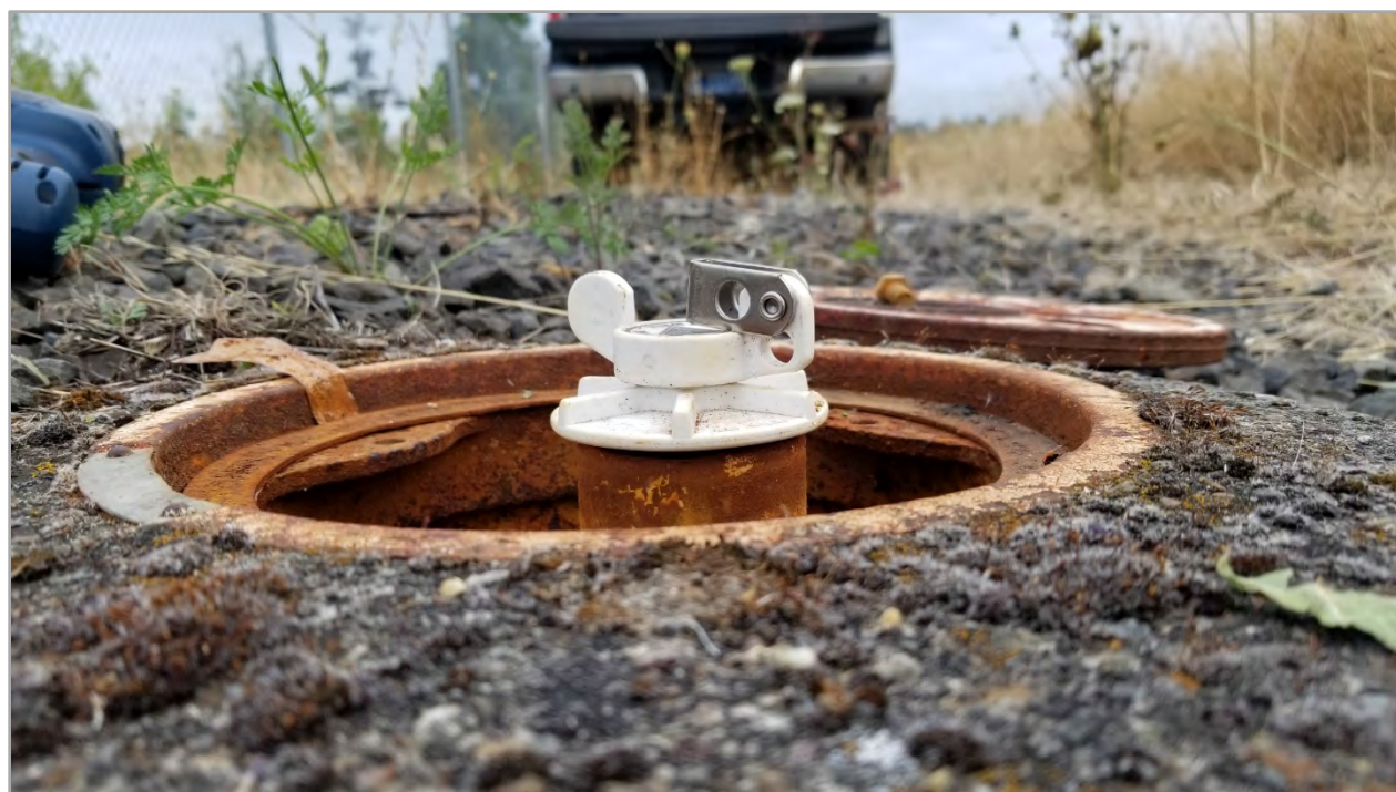
Photograph A16: MW-59s well casing and cap sticking above rim of well box prior to trimming (August 2019).
