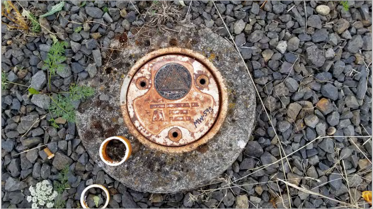
Photograph A17: Properly seated well box lid for MW-59s following trimming of the well casing by 2.125 inches (August 2019).
