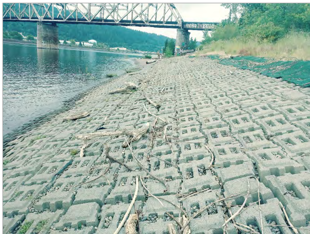
Photograph C24: Same area after shiny-leaf geranium removal (June 2019).
