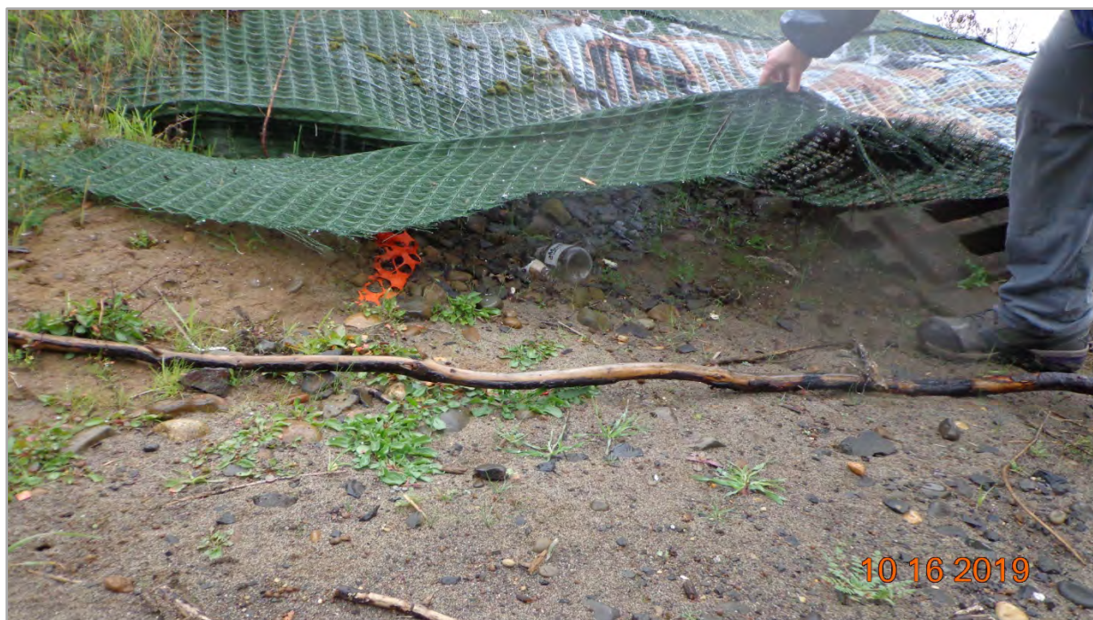
Photograph A19: Area of sand erosion under TRM along walking path near MW-37 well cluster (October 2019).
