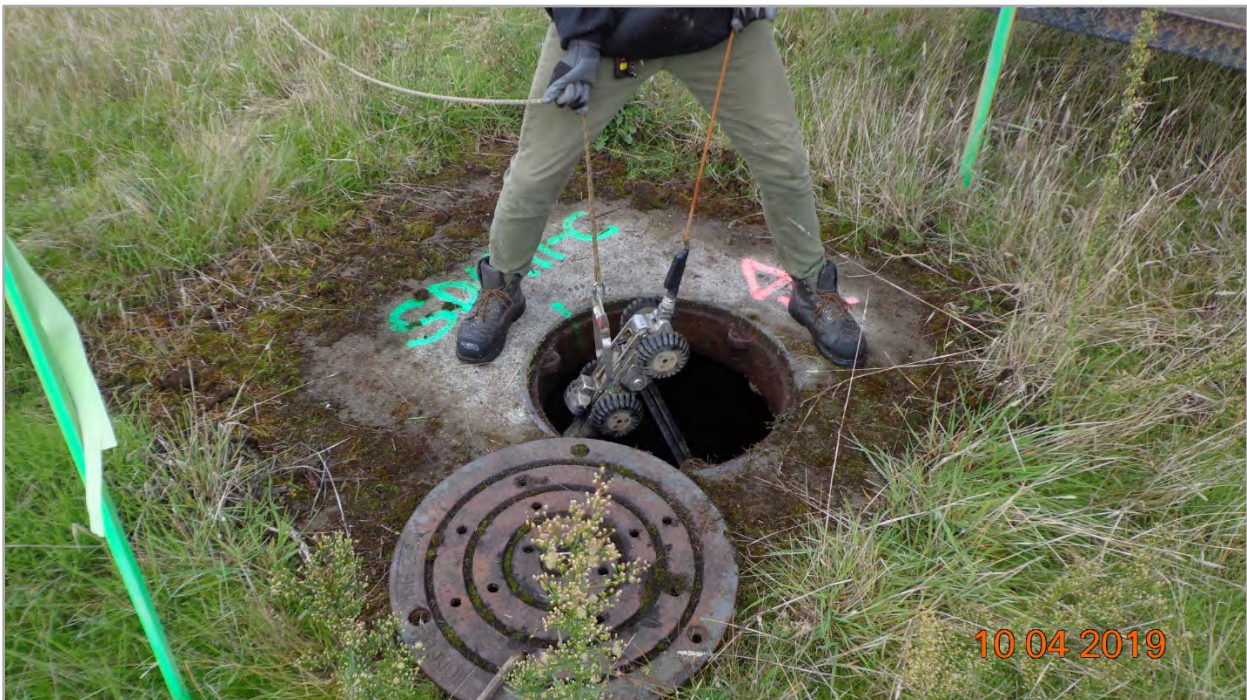
Photograph A18: Video inspection of the storm sewer using a robotic crawler. Crawler is being lowered into manhole SDMH-C (October 2019).
