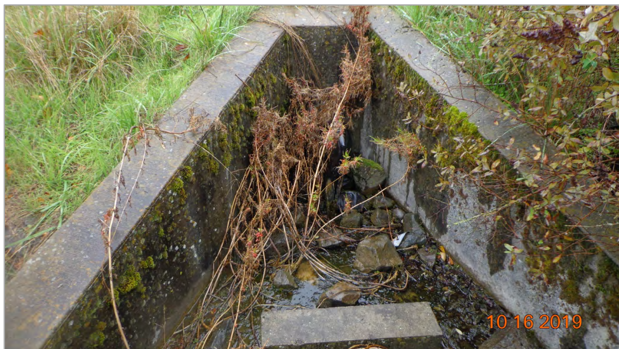
Photograph A20: Water drainage of less than 1 gallon per minute from the storm sewer outfall (October 2019).
