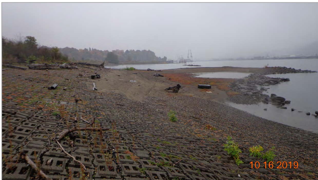
Photograph A21: Willamette River Shoreline during low tide in the vicinity of MW-39 well cluster facing southeast (October 2019). Driftwood and several items of trash visible, including a heavy equipment tire. Cover gravel washed down from the upper slope of the ACB is visible lower on the ACB slope.
