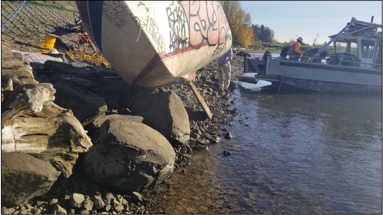
Photograph A17: Cutting of the fin keel on the derelict vessel to allow for removal of the vessel and trailering for transport to a disposal facility. View facing southeast (December 2021).
