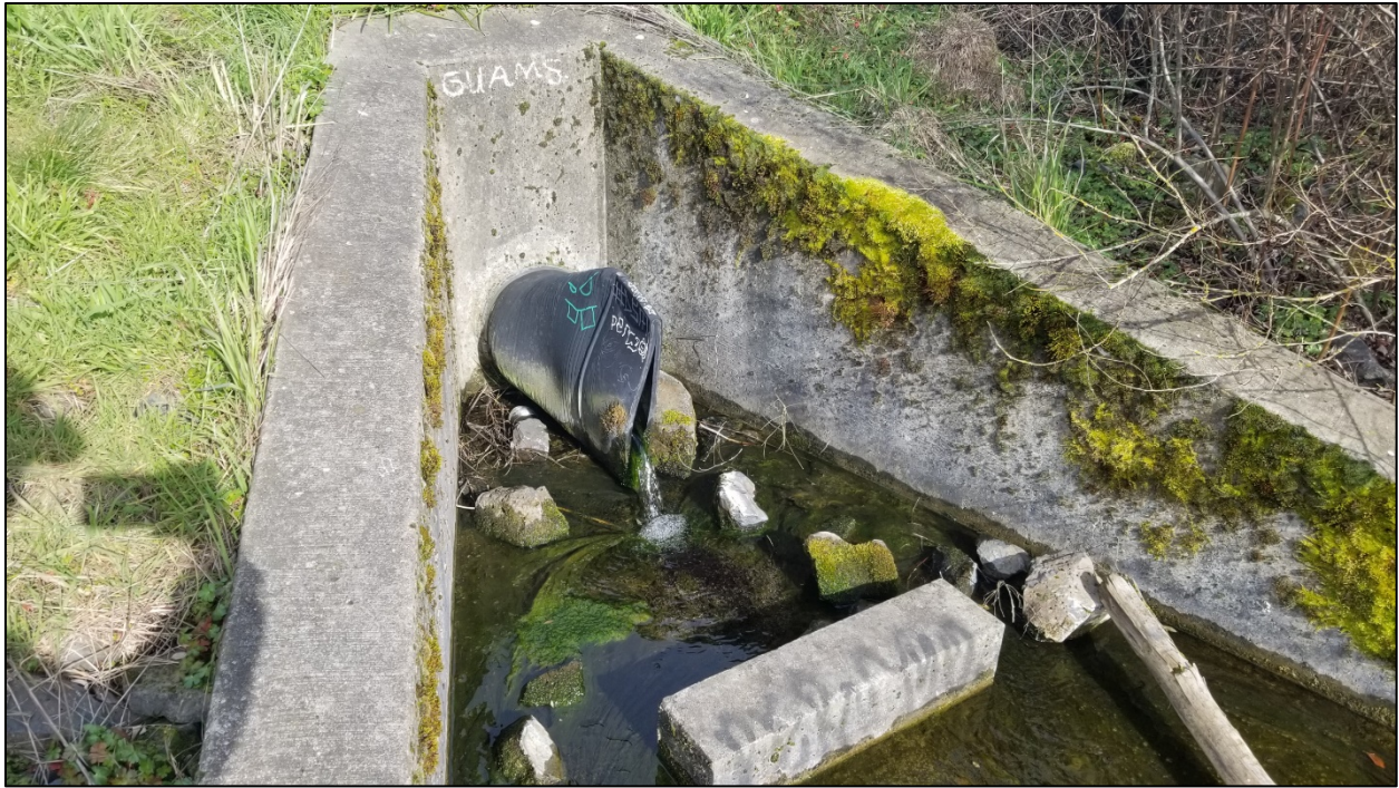
Photograph 3: Stormwater outfall with approximately 5-8 gpm of flow. View facing southeast.
