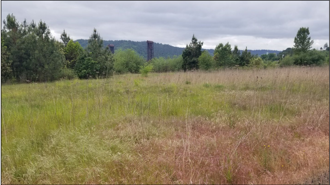
Photograph A9: Soil cap condition in southeastern quadrant of soil cap during the second quarter site inspection (May 2021).
