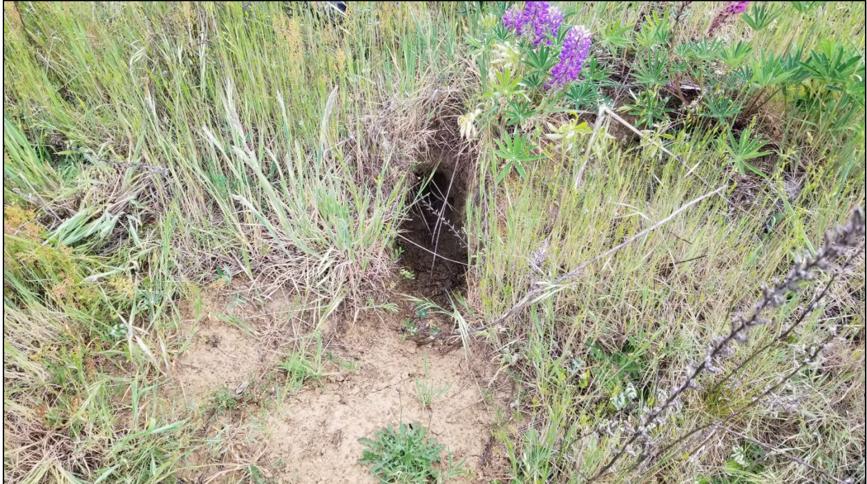
Photograph A8: Animal burrow in soil cap near MW-48s (May 2021).
