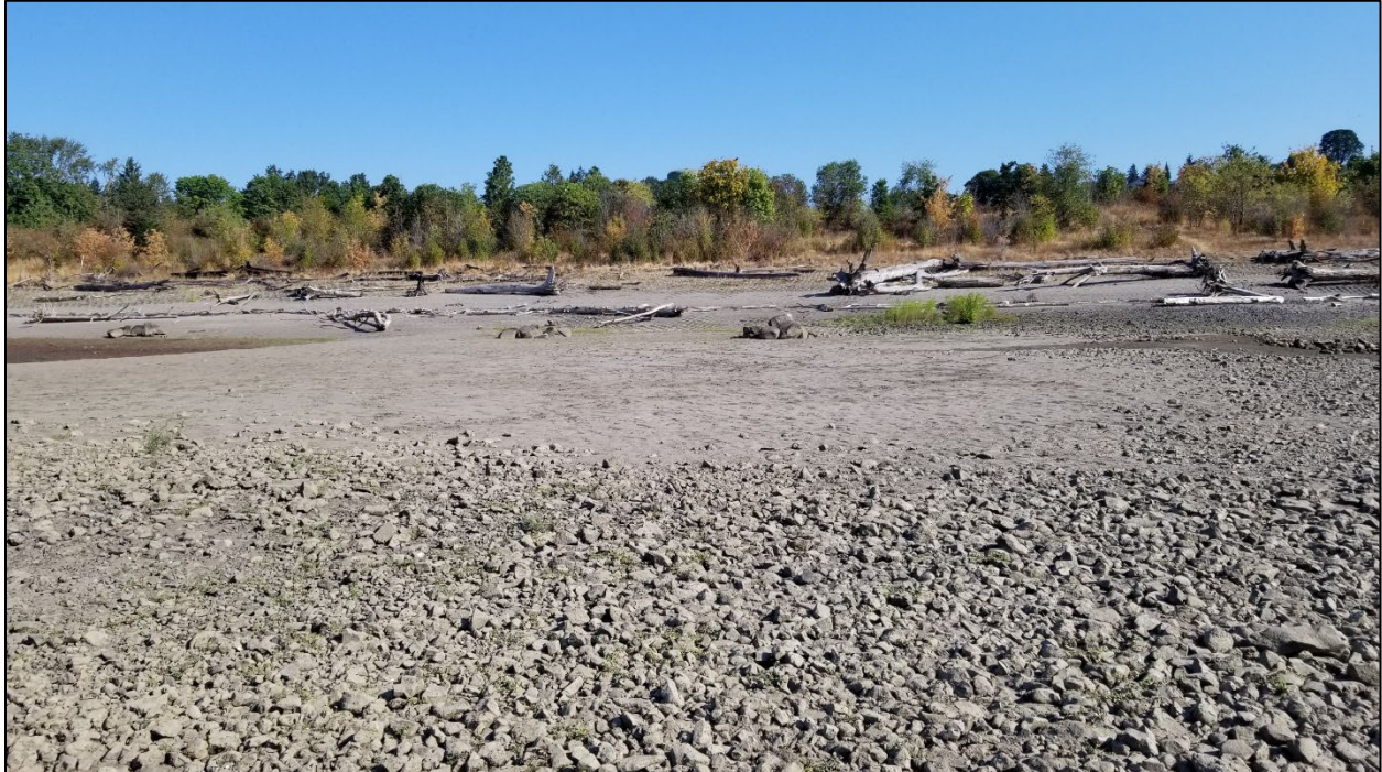
Photograph A16: Exposed sediment cap in intertidal zone during low river level conditions. View facing northeast (September 2021).
