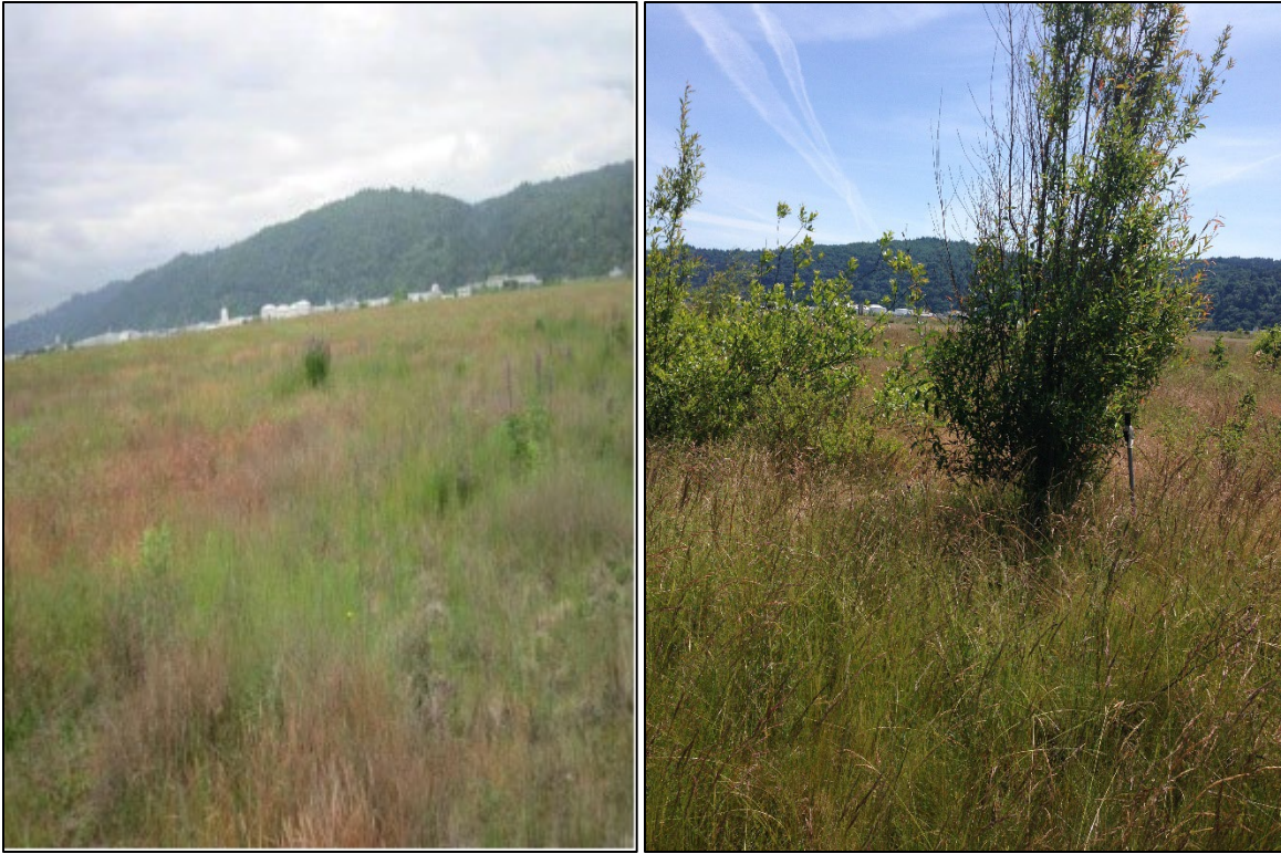
Photograph C1: Earthen cap and drainage swale in the foreground with the impermeable cap in the background. Taken looking south from Photograph Station 1 comparing baseline and conditions in 2014. (Left - June 2011, Right - June 2014).
