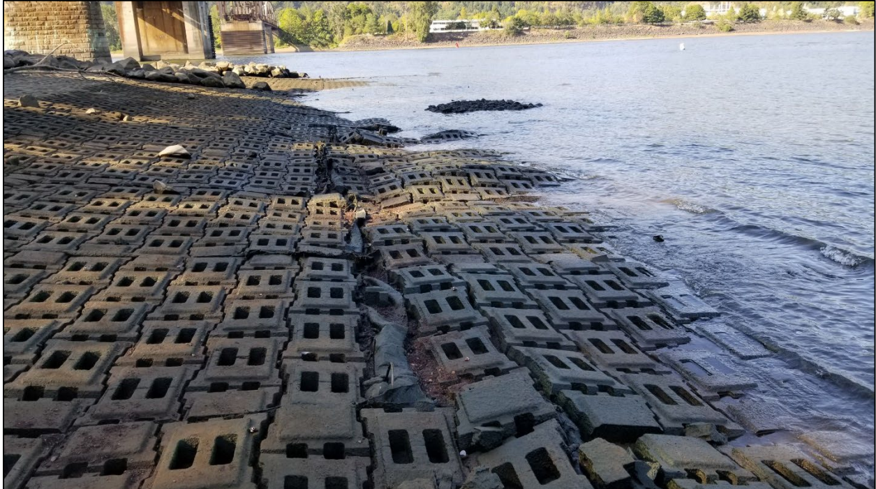
Photograph A14: Low river level and low tide conditions showing unconformities of the ACB in Willamette Cove. View facing west (September 2021).
