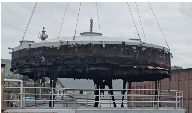
Crane removal of the damaged lid
