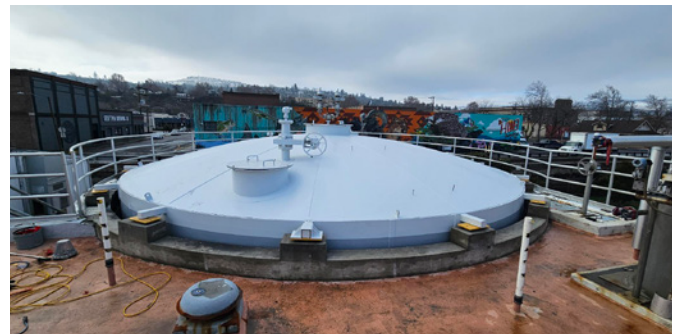
Repaired digester lid
