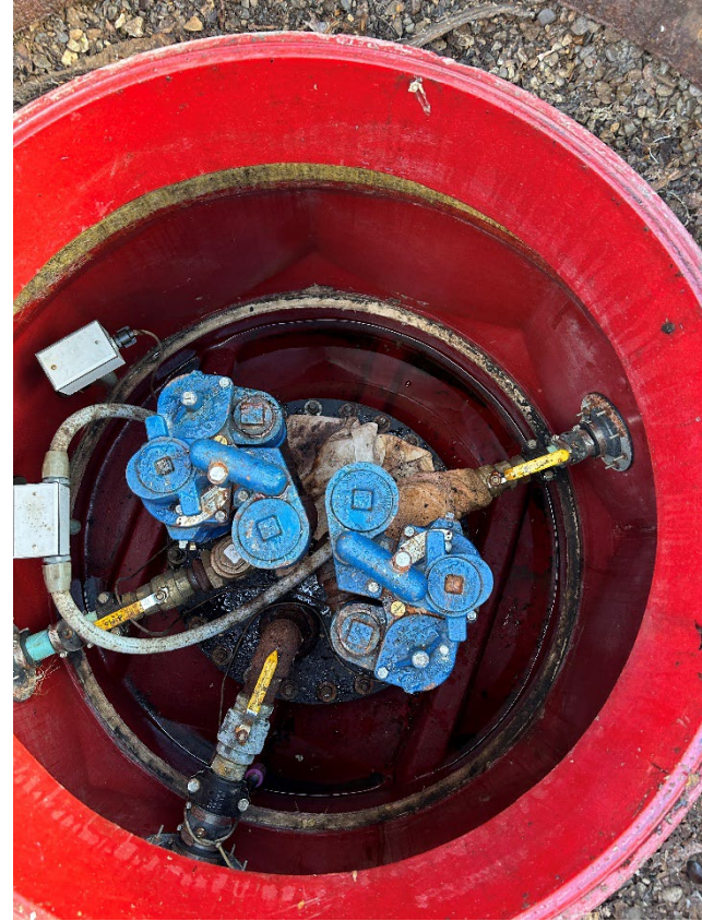
6: Transition sump with water present
