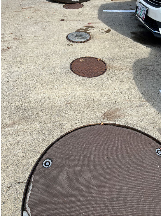
5: Tank nest looking north
