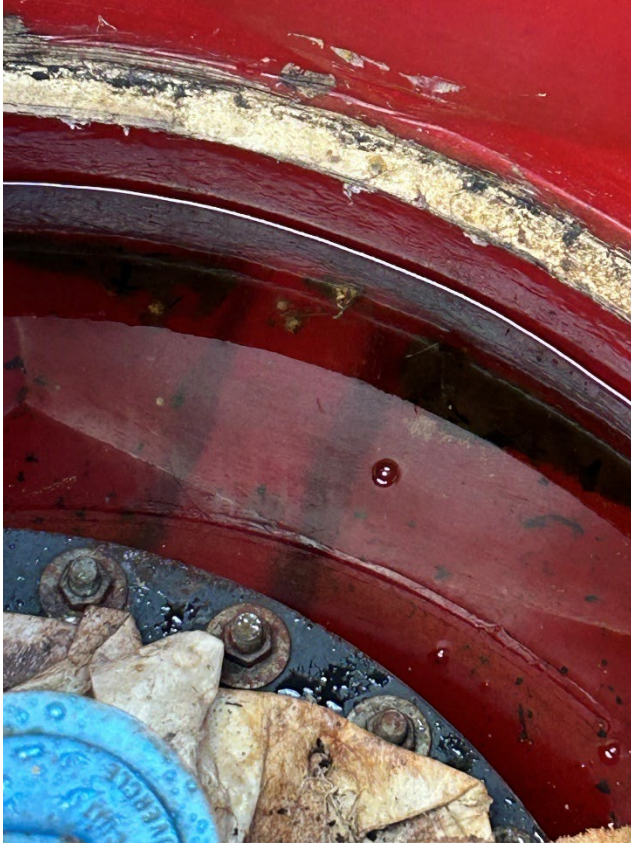
7: Water in transition sump
