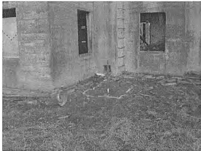
SW corner of building
