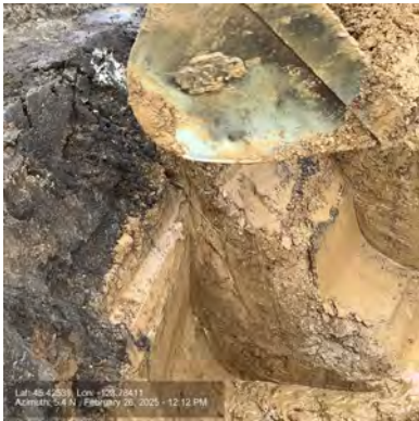
Picture taken at: 12:31 Caption: west sidewall at 8-9 feet bgs (before water inundates). Latitude: 45.42539 Longitude: -123.78411
