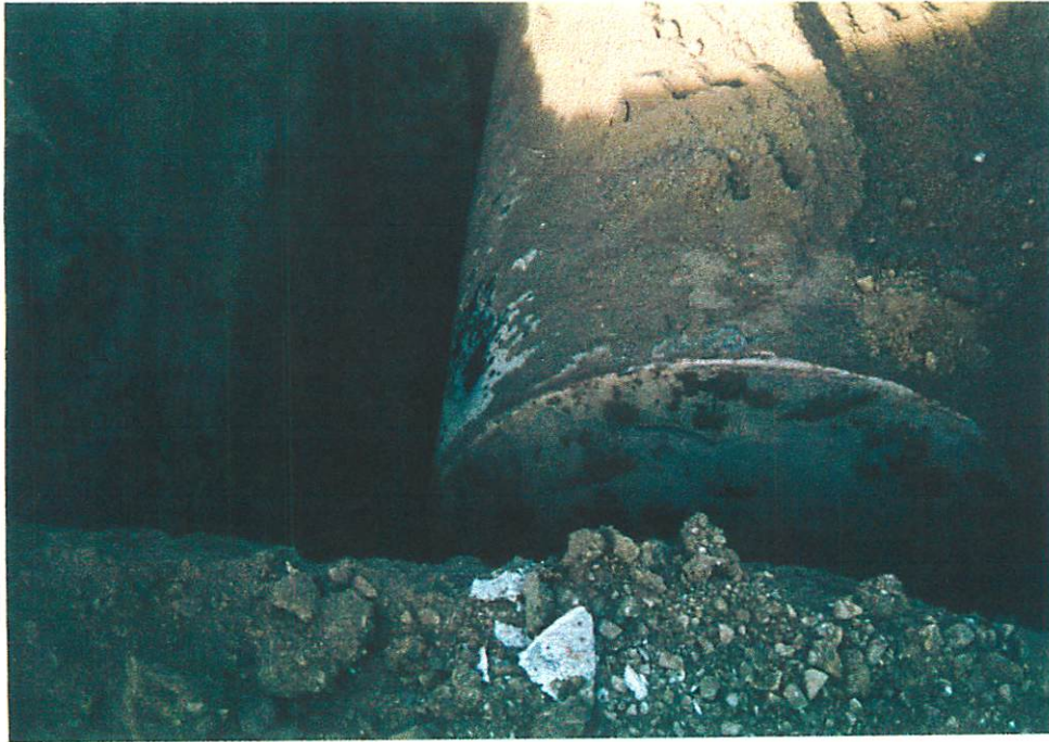
East end of tank prior to removal
