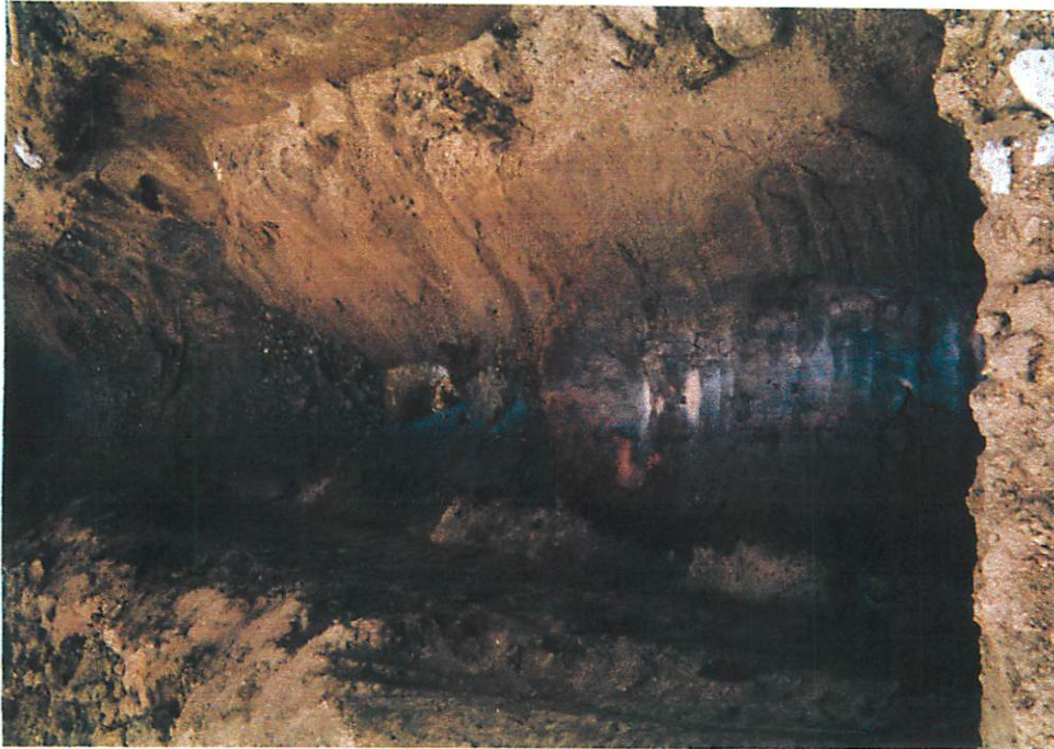
Bottom of excavation prior to removal of contaminated soil
