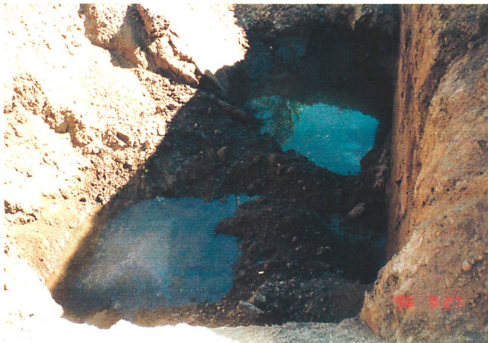
Bottom of excavation 24 hours after purging water
