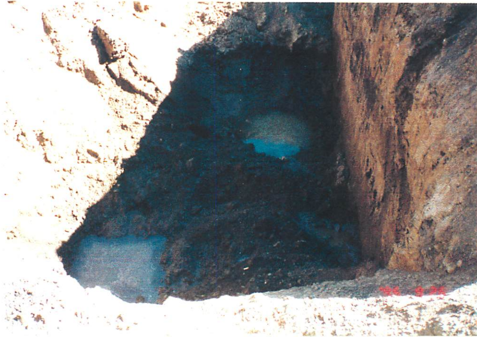
Bottom of excavation immediately after purging water
