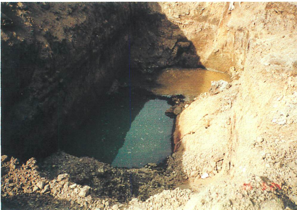
Bottom of excavation after contaminated soil removal
