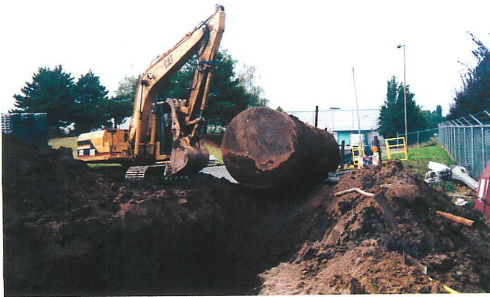
Tank temporarily placed at west end of excavation
