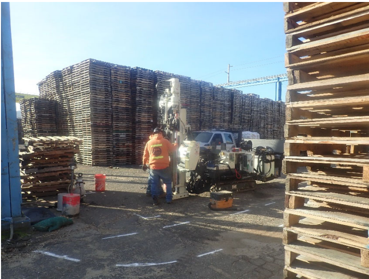
Utilizing direct-push rig outfitted with hollow stem auger to advance boreholes for monitoring well installation (MW01 location shown).
