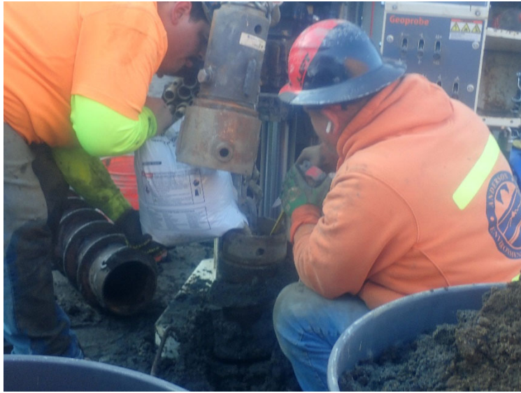
Pouring sand pack around MW02.
