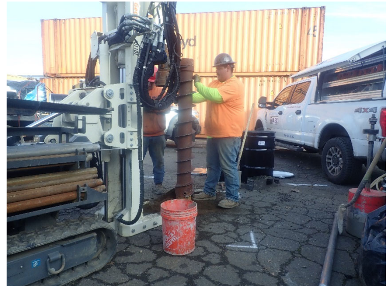
Installing MW02 in the southwest portion of site.
