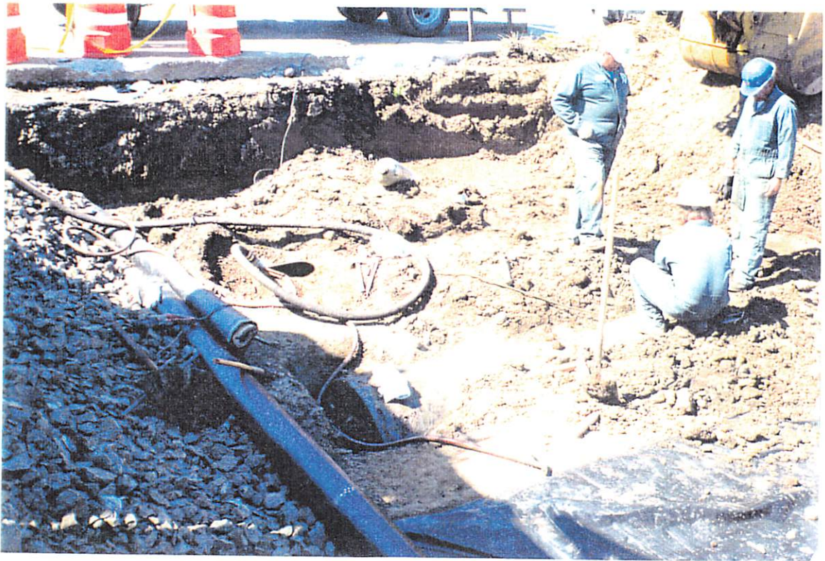
UST DECOMMISSIONING - VIEW TO THE SOUTH
