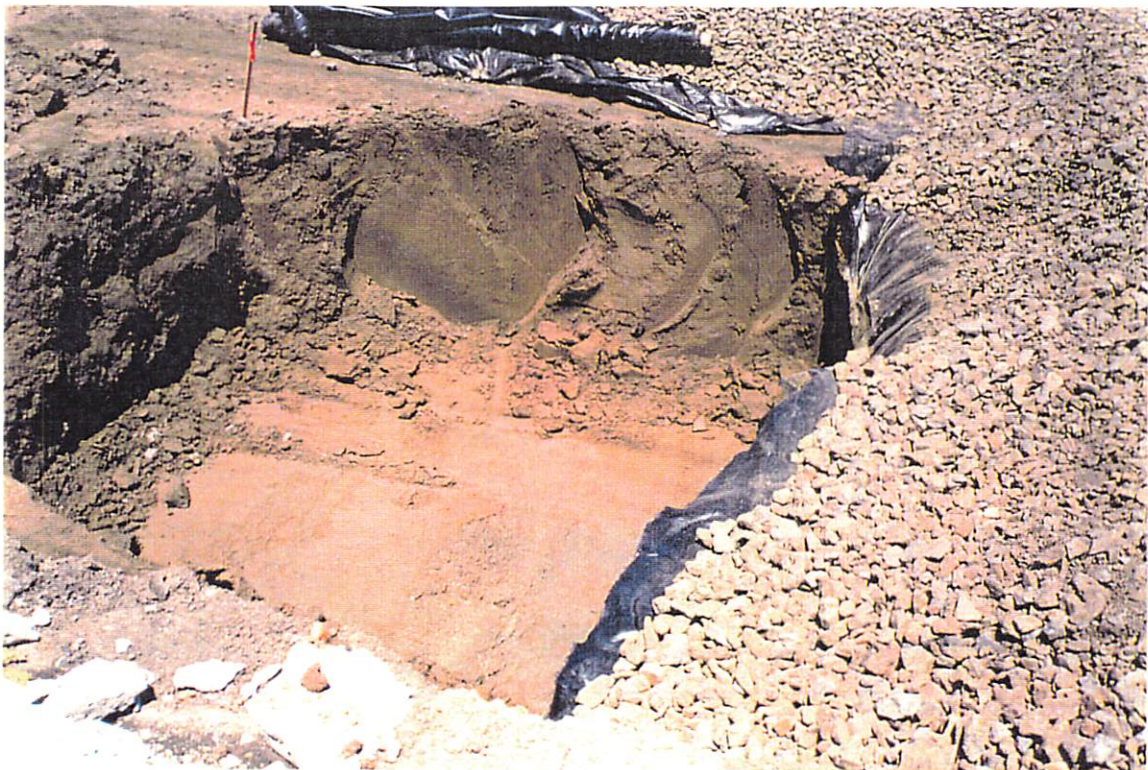
UST EXCAVATION EXCAVATION LIMITS ON 7/05/96
