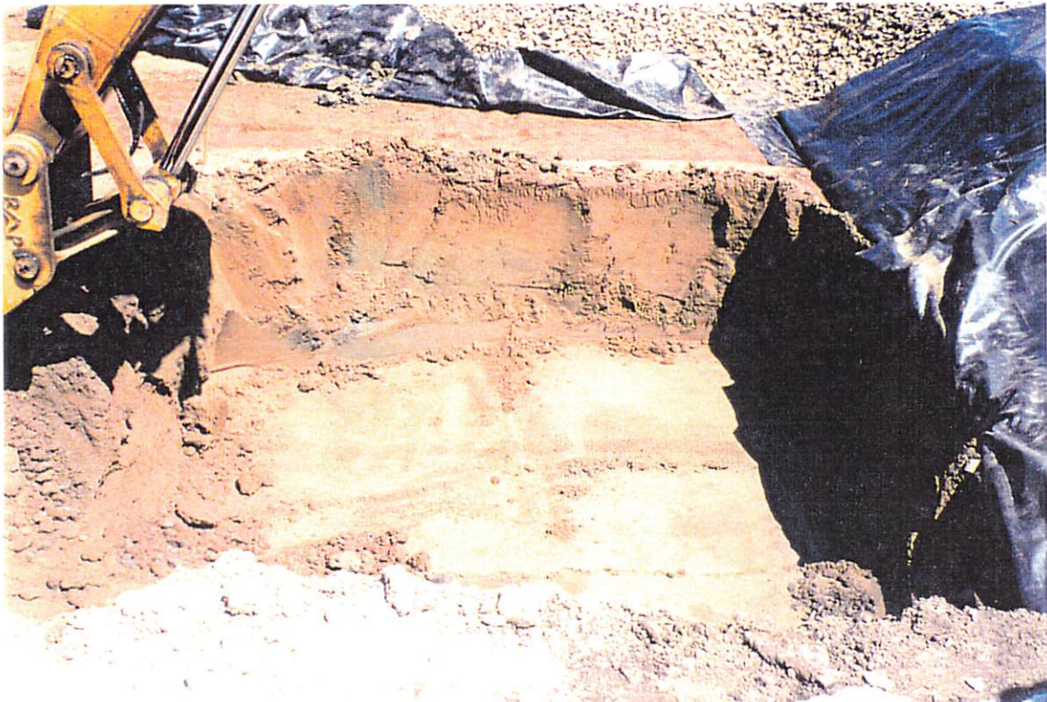
UST EXCAVATION AFTER REMOVAL OF USTs & DURING REMOVAL OF CONTAMINATED SOIL
