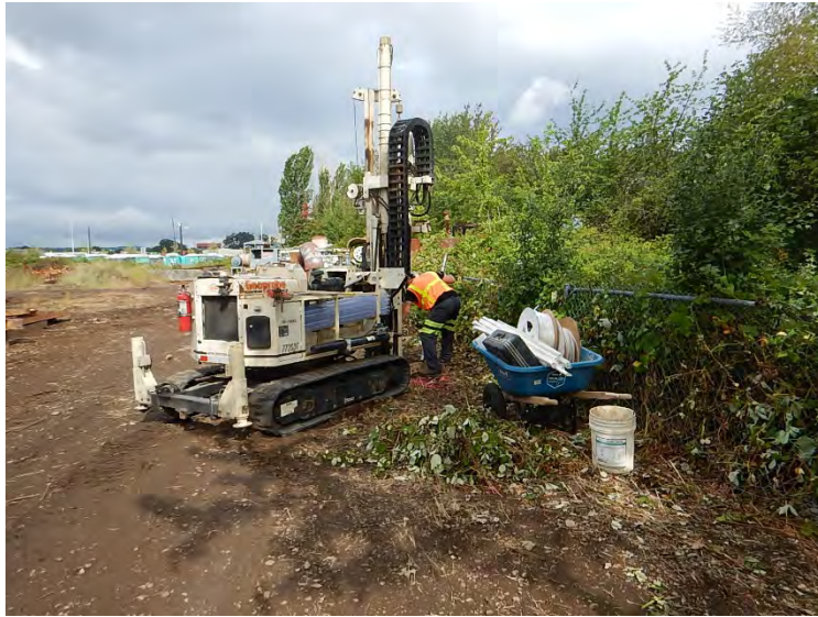
View looking west during drilling of EB01. The fence surrounds the onsite pond (out of sight) to the right.
