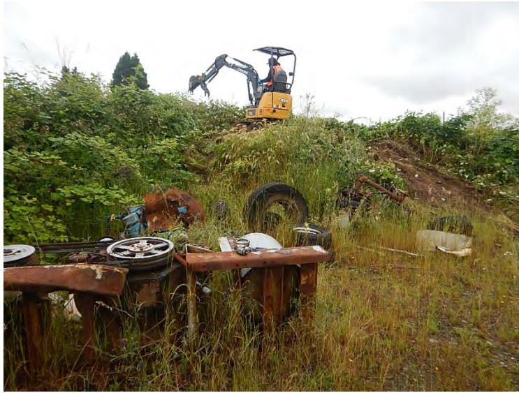
A mini excavator was used to collect an incremental sample from soil pile SP01 located near the southwest corner of the site.
