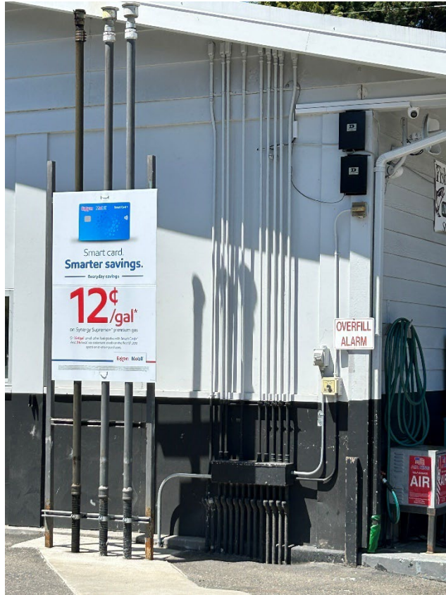
3: Overfill alarm and vapor vent caps
