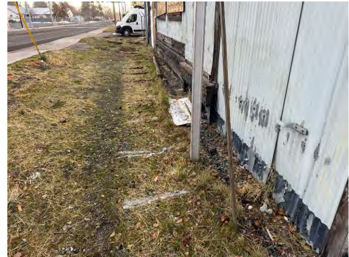
Continued dripline sampling along Warehouse Building. (facing south)
