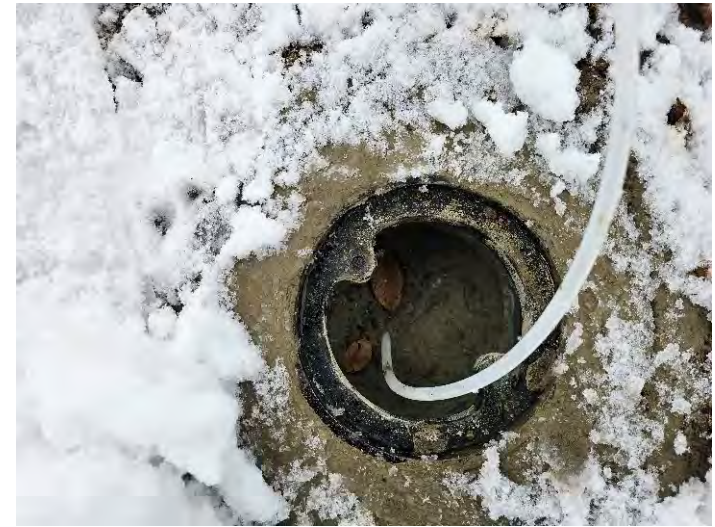
Concrete successfully set at VP-1.
