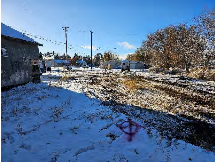
Boring location TMW-2/BH-2. (facing south)
