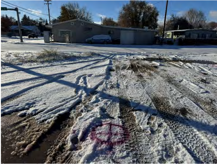
Boring location TMW-6/BH-6. (facing south)
