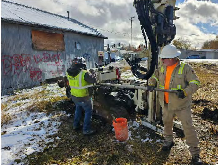
Extracting core at TMW-2/BH-2. (facing southeast)
