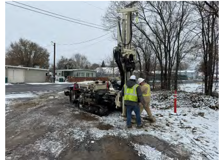
Drilling at TMW-5/BH-5. (facing south)
