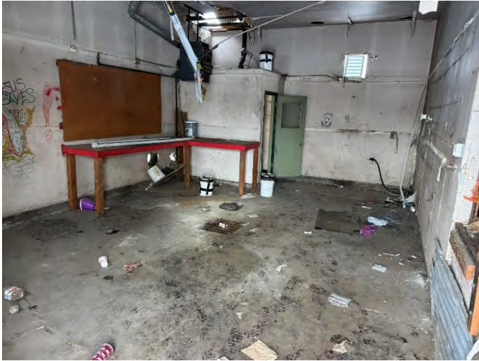
Interior of Warehouse Building.
