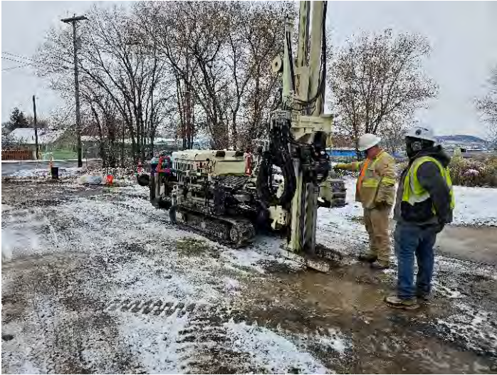
Drilling at TMW-6/BH-6. (facing southwest)
