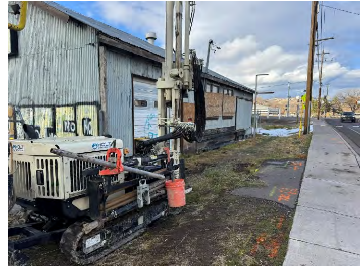
Drilling at TMW-3/BH-3. (facing north)
