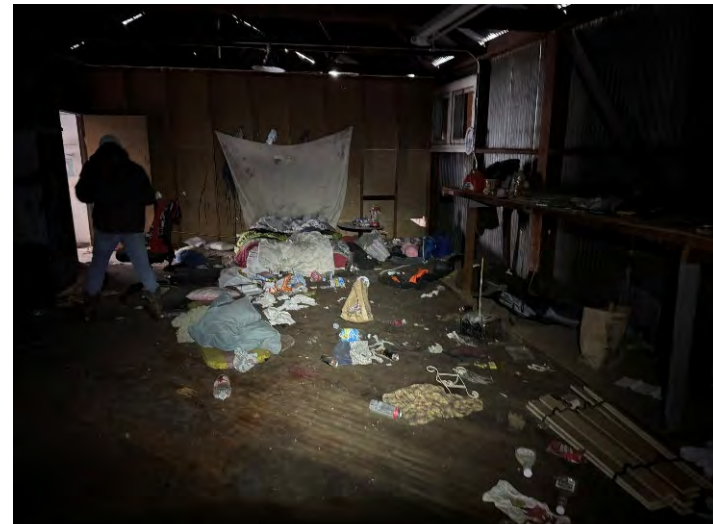
Interior of Warehouse Building.
