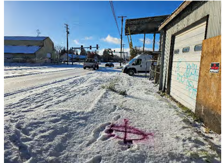
Boring location TMW-3/BH-3. (facing south)
