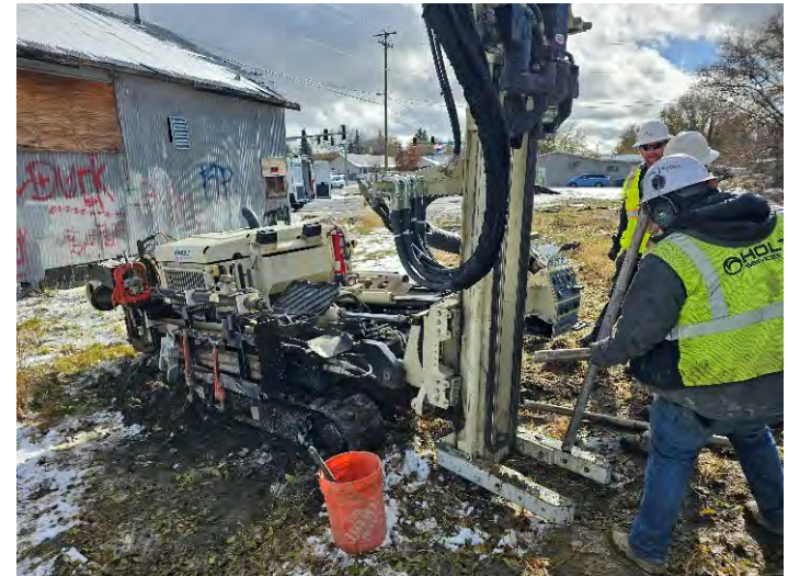
Drilling at TMW-2/BH-3. (facing southeast)
