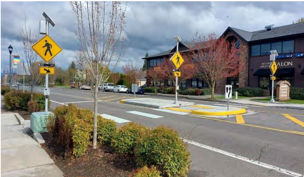
Figure 20. Typical Enhanced Pedestrian Crossing with a Refuge Island
