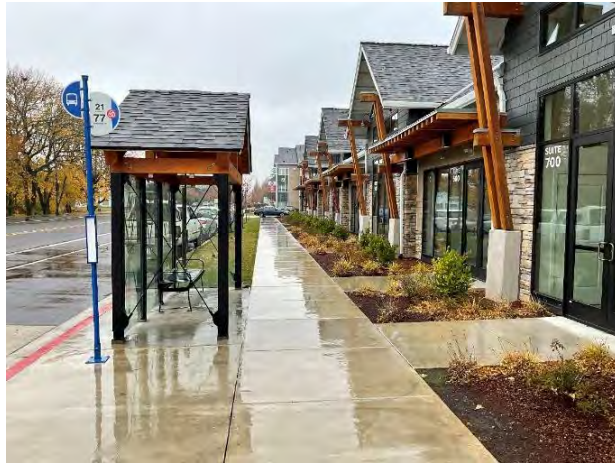
Image 8: TriMet Stop in Wood Village
