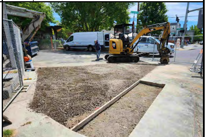
Photo #6: Site Restoration
