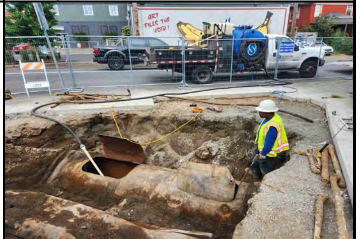
Photo #4: Decommissioning and Cleaning
