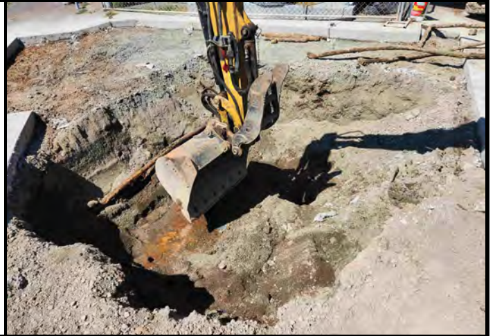
Photo #2: Initial Excavation
