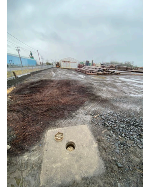
Image 1: French Drain cleanout (looking West) Image 2: French Drain cleanout (looking South)
