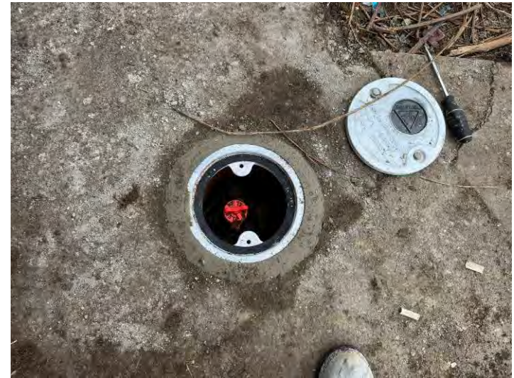
MW-5 completed monitoring well.
