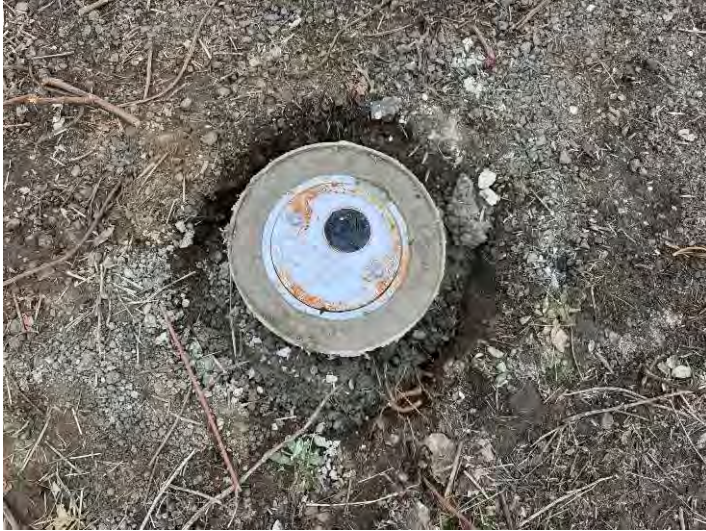
MW-6 completed monitoring well.
