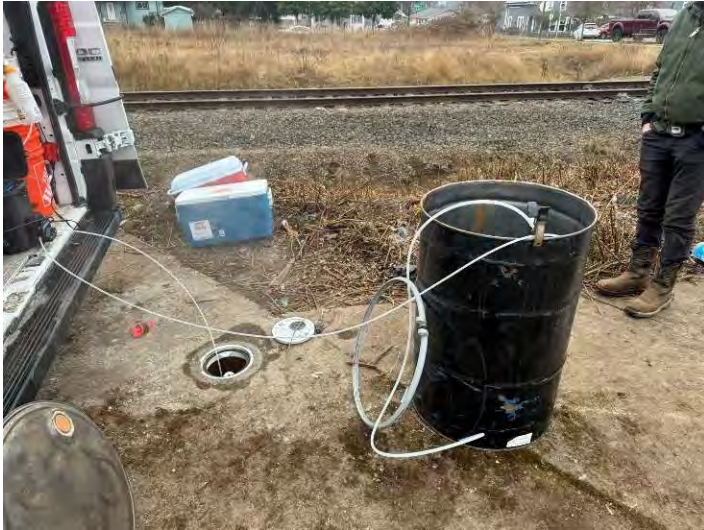
Developing MW-5 (facing south).
