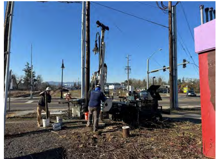
Drilling crew installing MW-6 (facing west).
