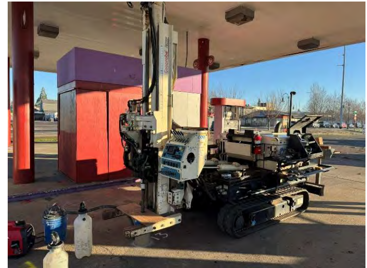
Concrete coring set up on the drill rig (facing northeast).
