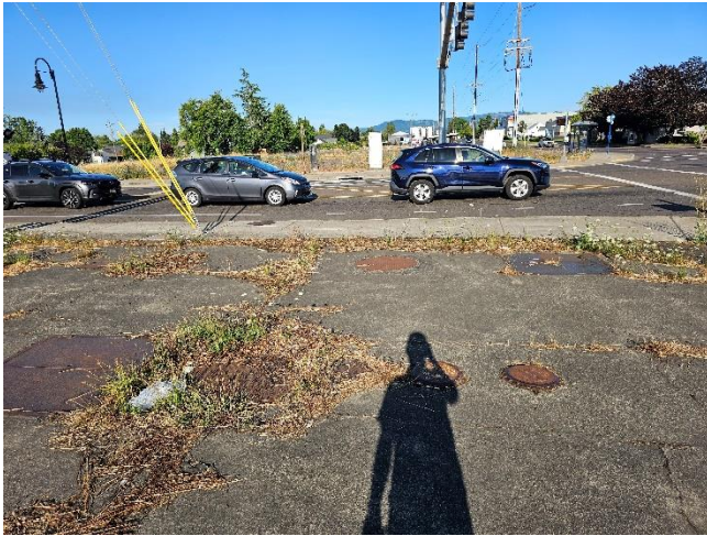
10k gallon (furthest away) and 3k gallon UST (facing S 10 th Avenue)
