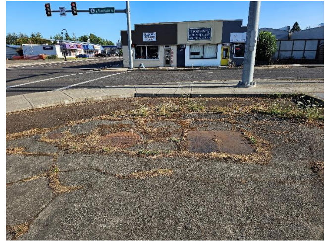
8K unleaded UST (facing Baseline Street).
