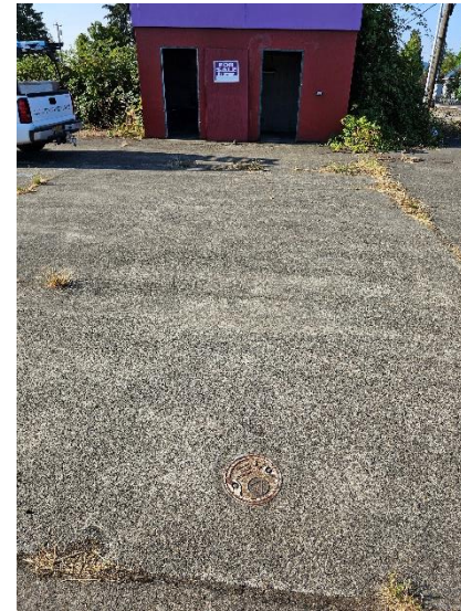
Monitoring well in front of office/bathroom shed.
