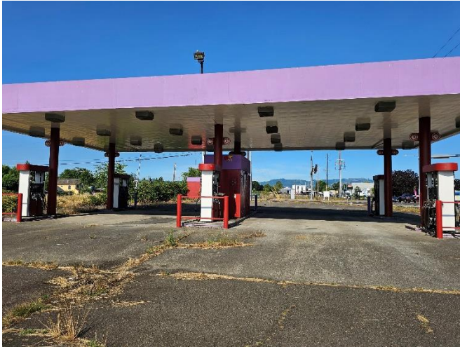
Fuel canopy/pump islands facing N 10 th Avenue.
