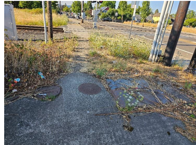
4k gallon Super UST (facing railroad, adjacent to bathroom/office shed).
