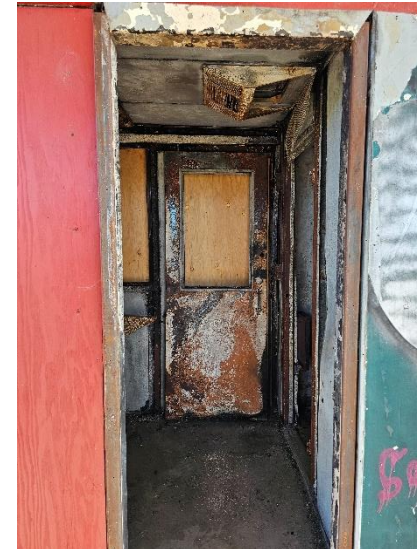
Entrance of kiosk area, standing from outside.
