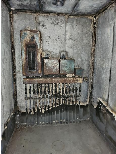
Burnt power box to the right of kiosk area.
