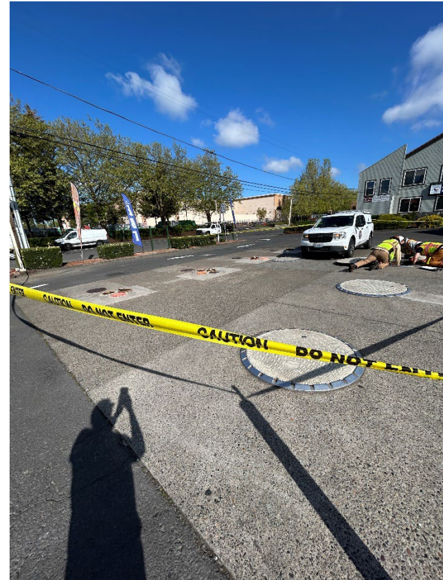
2: Tank nest looking north
