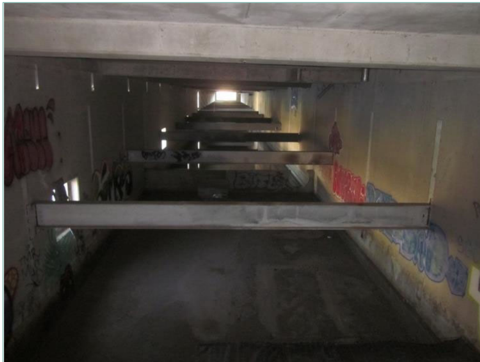
Photo 6: View of inside Pipe Tunnel.
