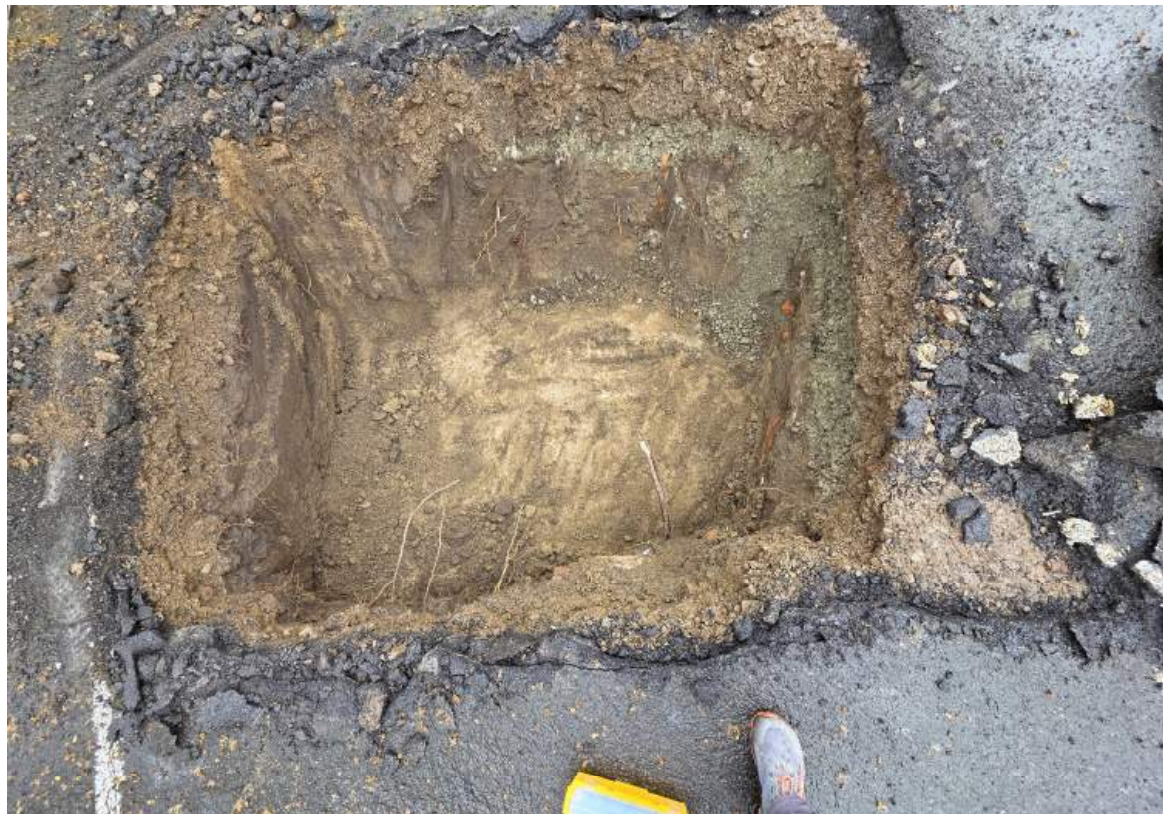
AERIAL VIEW OF THE REMEDIAL EXCAVATION LIMITS FOLLOWING REMOVAL OF THE LEAD-IMPACTED SOIL.
