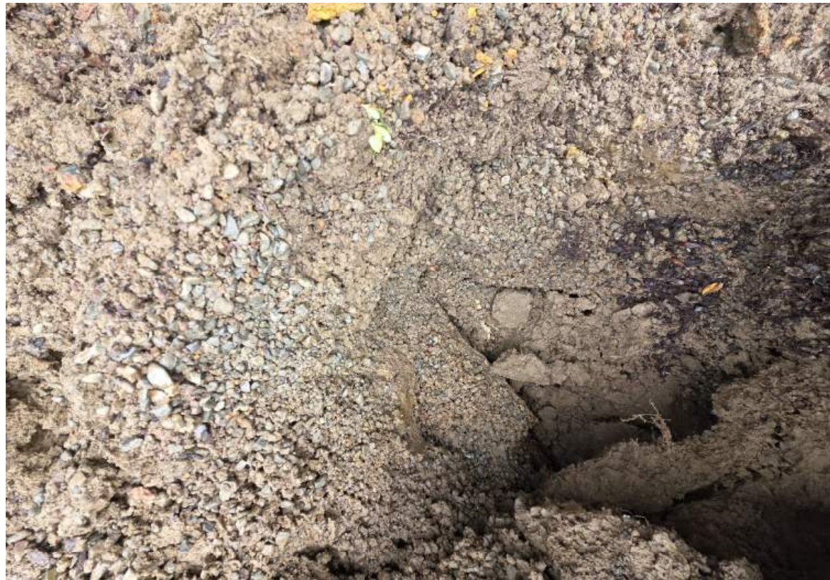
VIEW OF THE PREVIOUSLY-DECOMMISSIONED UST (GEOPHYSICAL ANOMALY). THE UST HAD BEEN CUT OPEN AND FILLED IN-PLACE WITH PEA GRAVEL.
