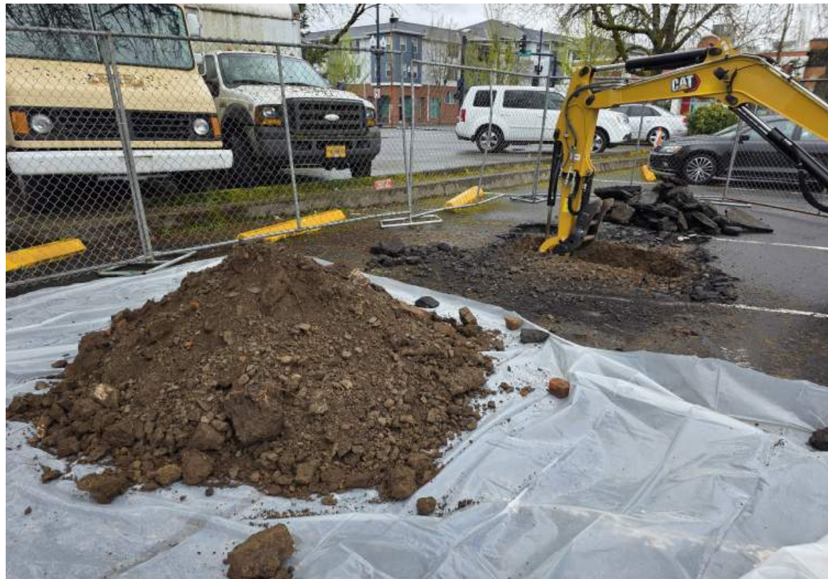
REMEDIAL EXCAVATION OF LEAD-IMPACTED SOIL AT THE PROPERTY. PHOTO TAKEN FACING WEST. THIS SOIL WAS DISPOSED OF AT THE WM HILLSBORO LANDFILL.
