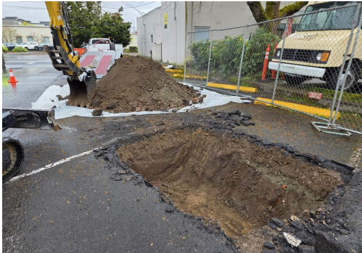
REMEDIAL EXCAVATION OF LEAD-IMPACTED SOIL AT THE PROPERTY. PHOTO TAKEN FACING EAST. THIS SOIL WAS DISPOSED OF AT THE WM HILLSBORO LANDFILL.
