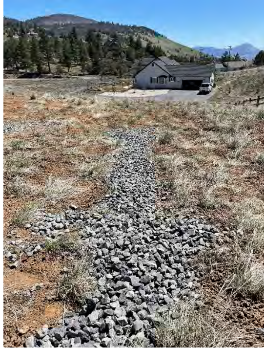
Swimming Pool Repository – Before/after view of repaired gully on Parcel AG; the gully was armored/backfilled with quarry rock to prevent additional erosion.
