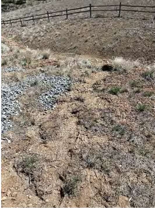
Memorial Park Repository – Before/after view of repaired gully along Hunters Ridge Road on Parcel MBK-D; the gully was armored/backfilled with quarry rock to prevent additional erosion.
