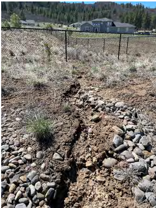
Memorial Park Repository – Before/after view of repaired gully along Parcels MBK-D and P; the gully was armored/backfilled with quarry rock to prevent additional erosion.
