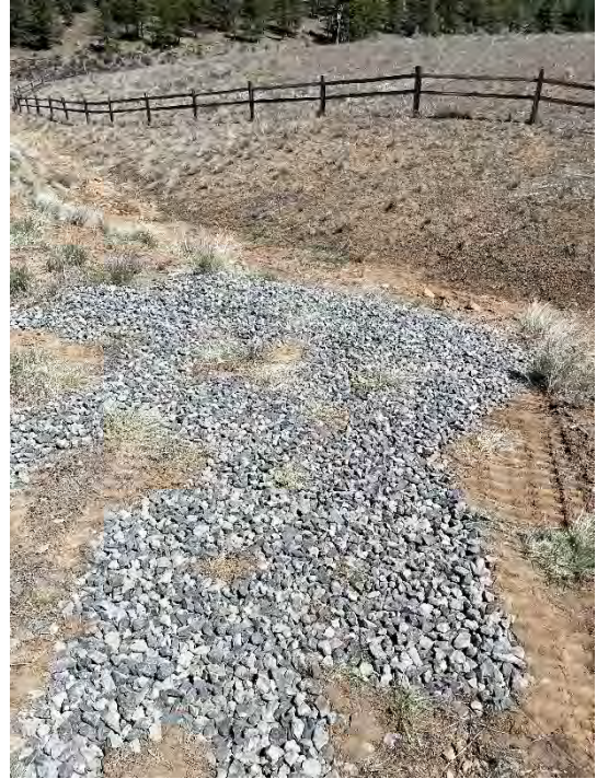
Memorial Park Repository – Before/after view of repaired gully along Hunters Ridge Road on Parcel MBK-D; the gully was armored/backfilled with quarry rock to prevent additional erosion.
