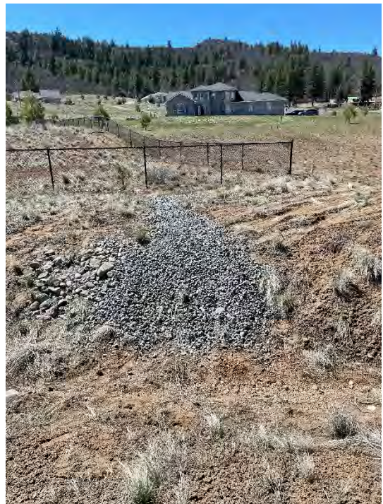
Memorial Park Repository – Before/after view of repaired gully along Parcels MBK-D and P; the gully was armored/backfilled with quarry rock to prevent additional erosion.
