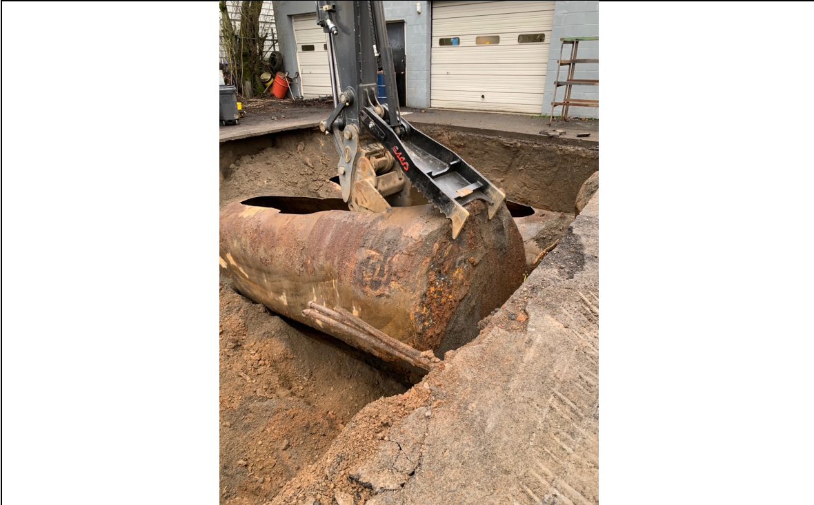
T1, T2, and T3 were then removed from the ground.
