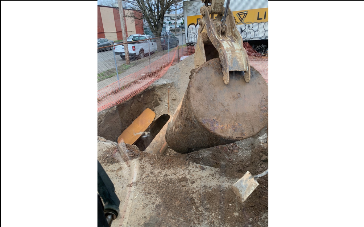
T4, T5, and T6 were then removed from the ground.
