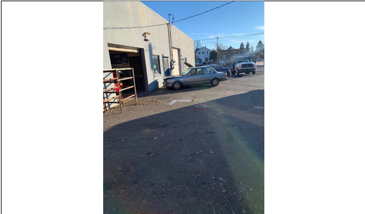
USTs were located in the parking lot located in the northwest portion of the site.
