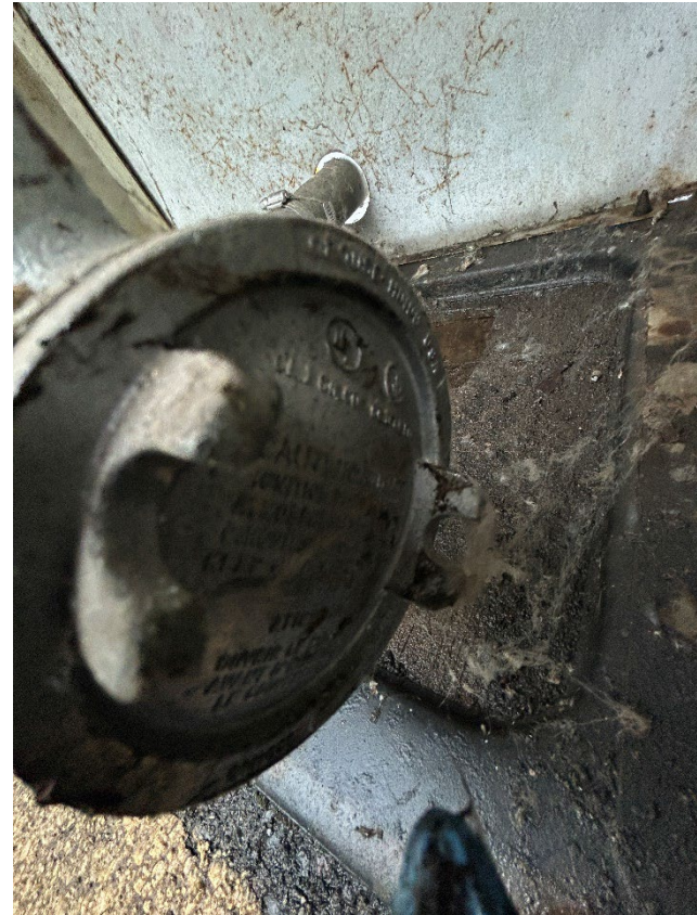
6: Check Valve for safe suction
