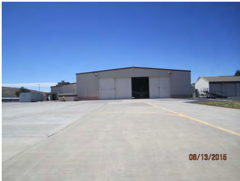
Photo 2: Hangar 333 from Apron Side
