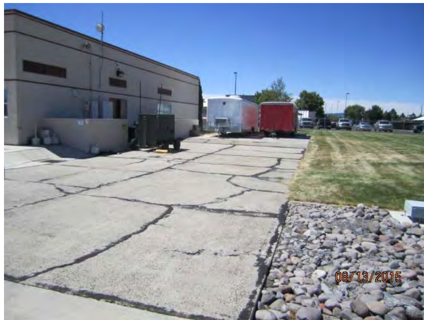
Photo 12: Area of Former Fire Station (grassy area) North of Current Fire Station
