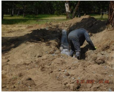
Tile Dewatering Drain, West End
