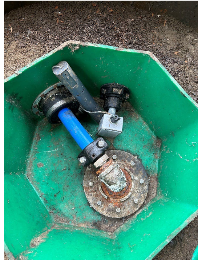
10: Transition sump with sensor
