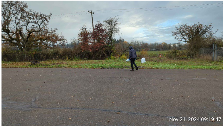
Before drilling, ENW conducted a geophysical survey to clear boring locations of utilities.
