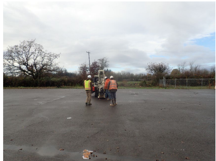
Temporary soil borings were advanced using a track-mounted DPT drill rig.
