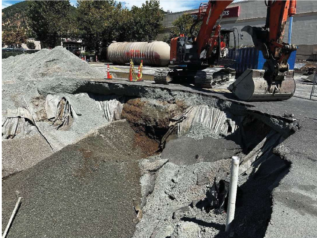
Figure 5. UST-E-6 east sidewall sample excavation.
