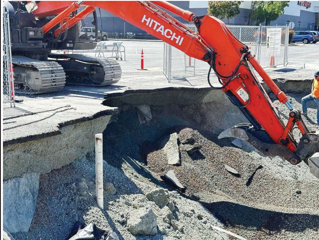
Figure 7. UST Excavation, southern sidewall sampling attempt.
