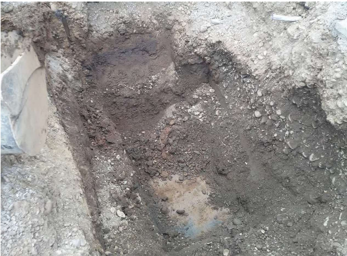
Used oil UST excavation prior to sample collection.
