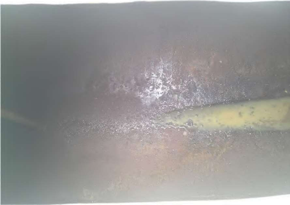
Gas UST post-cleaning – typical.
