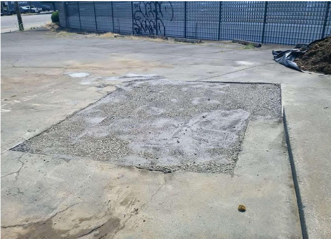
Used oil UST excavation following backfilling.
