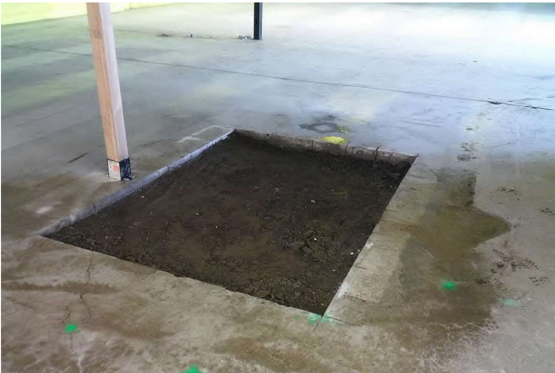
Kerosene or heating oil UST following backfilling.
