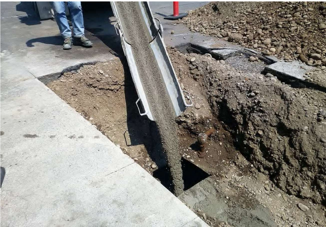
Filling of gas USTs with inert materiall – typical.
