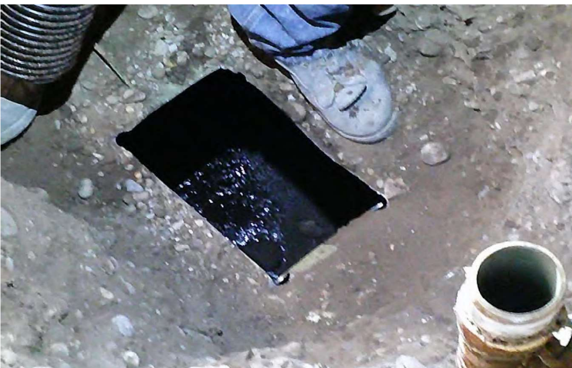
Kerosene or heating oil UST after cleaning.
