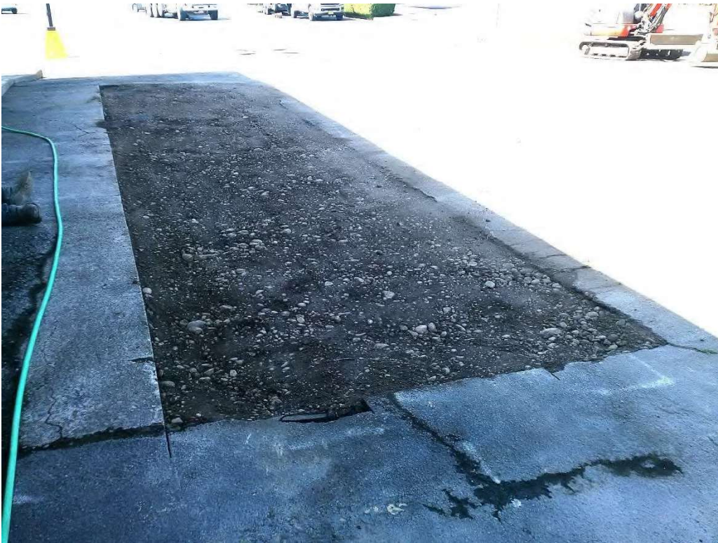
Gas UST area following excavation backfilling.
