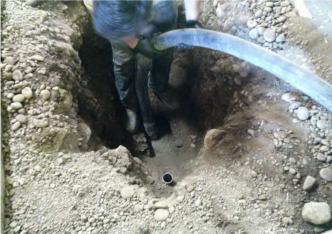
Filling kerosene or heating oil UST with inert material.
