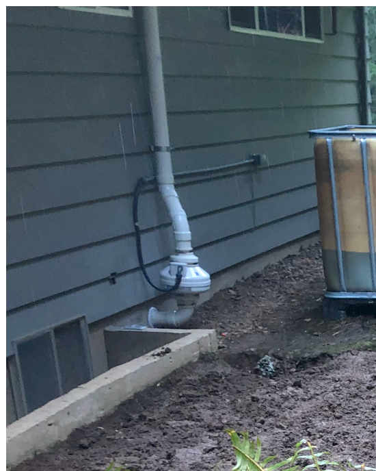
Photo 16. A vapor mitigation system was installed on the east side of the house. View is to the northwest.
