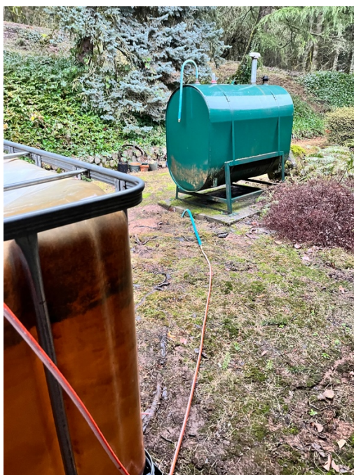
Photo 5. The AST contents were removed and product lines were transferred to a temporary AST for future use. View is to the southeast.
