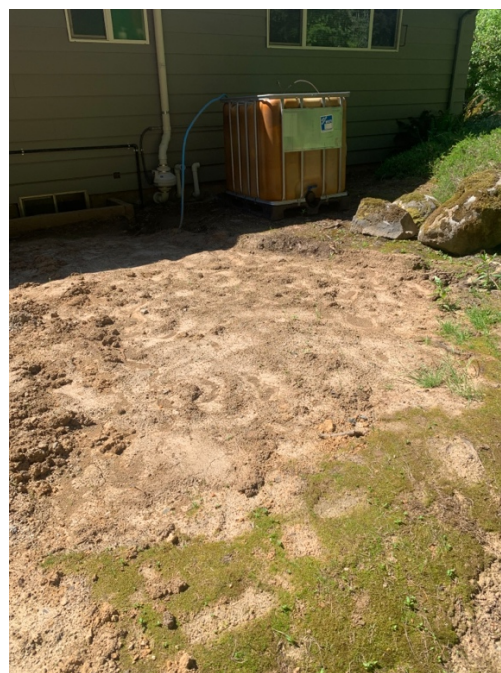
Photo 14. The excavation area was backfilled with gravel. View is to the west.
