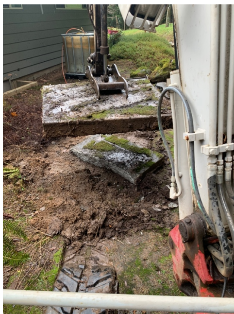
Photo 9. The concrete pad was removed. View is to the northwest.
