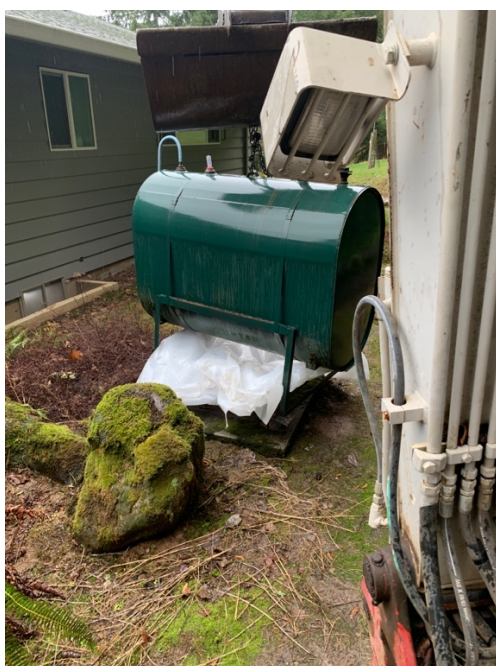
Photo 7. The AST was emptied and removed from the property. View is to the northwest.
