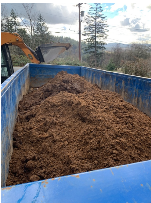
Photo 11. Contaminated soil was transported for proper disposal. View is of removed soil.
