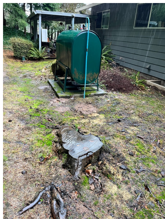
Photo 4. View of the AST and concrete pad. View is to the southwest.
