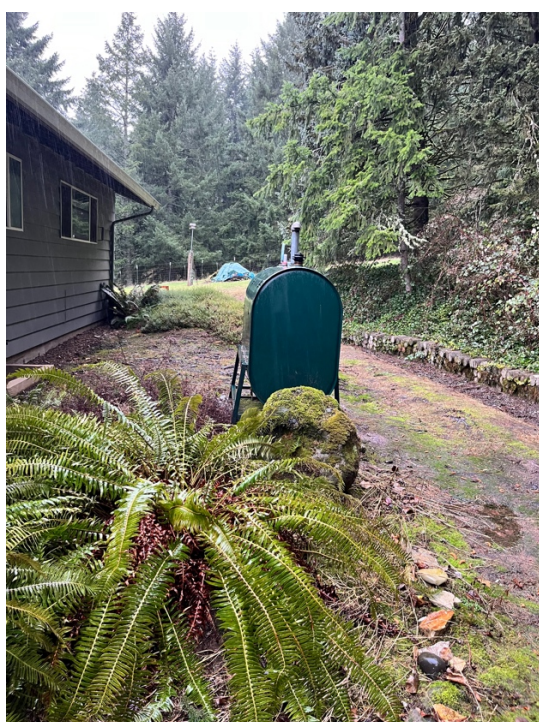
Photo 3. The AST was located east of the house. View is to the north.
