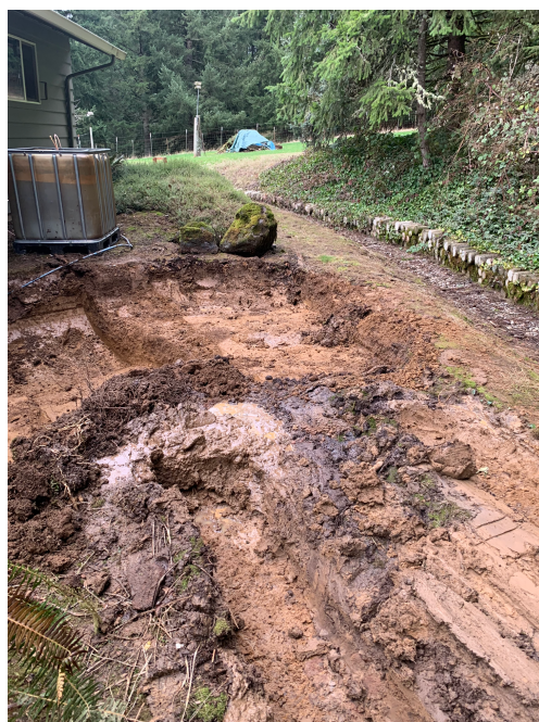
Photo 12. Excavation area. View is to the north.
