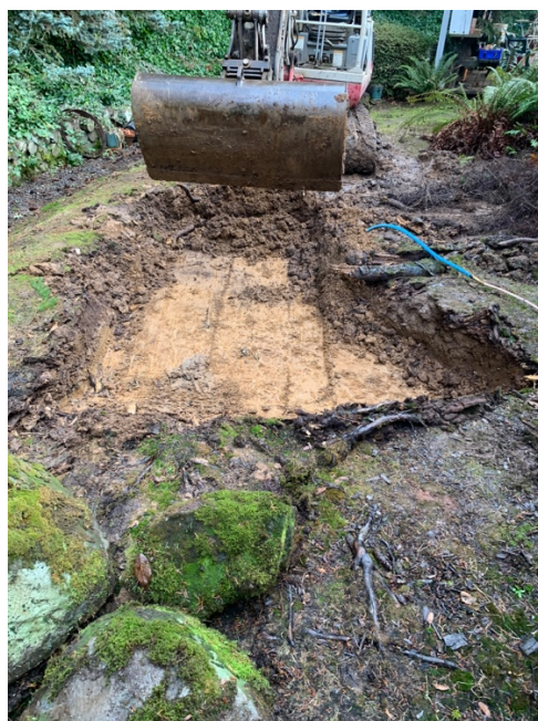
Photo 10. Contaminated soil removal began below the former AST location. View is to the south.
