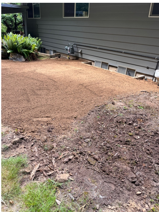
Photo 15. The former AST area was restored to grade with soil. View is to the southwest.
