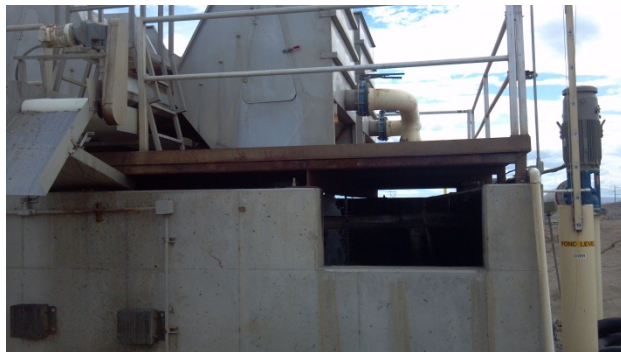
Figure 4. Vault structure showing a window for interchange with the atmosphere and screens above.
