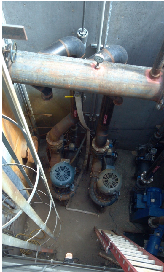
Figure 3. Pit dry side pumps for transport from pit to the vault.
