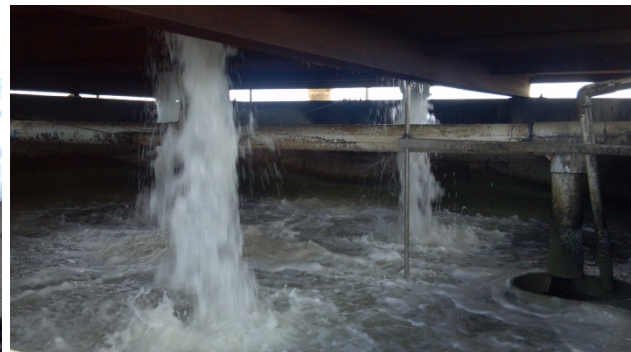
Figure 5. Interior of the vault showing frothy discharge from screens above.
