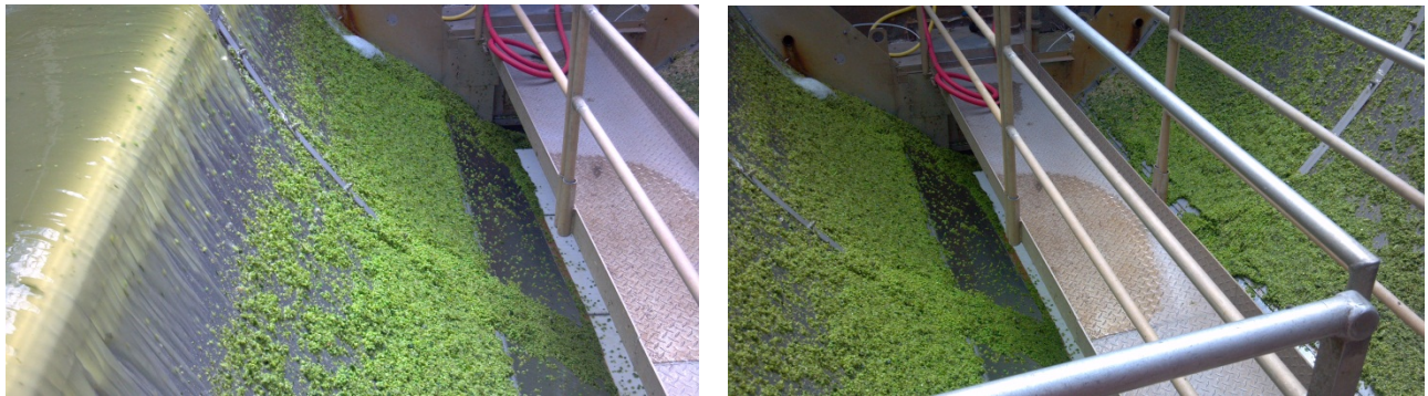
Figure 2. Screens to collect solids prior to the water storage pit at the Hermiston processing facility.
