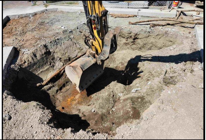
Photo #2: Initial Excavation
