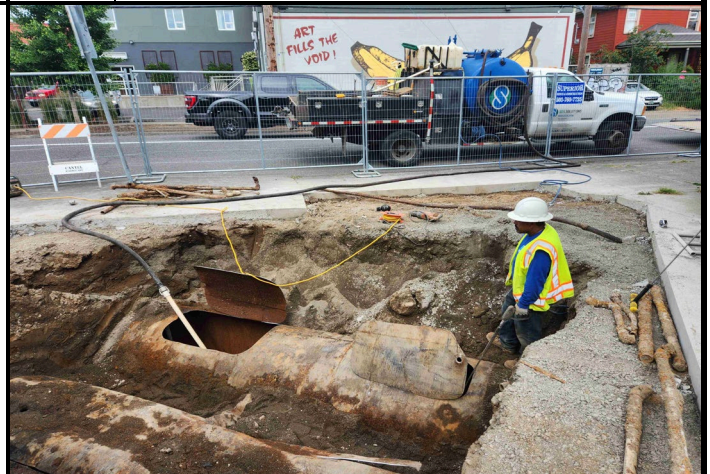
Photo #4: Decommissioning and Cleaning
