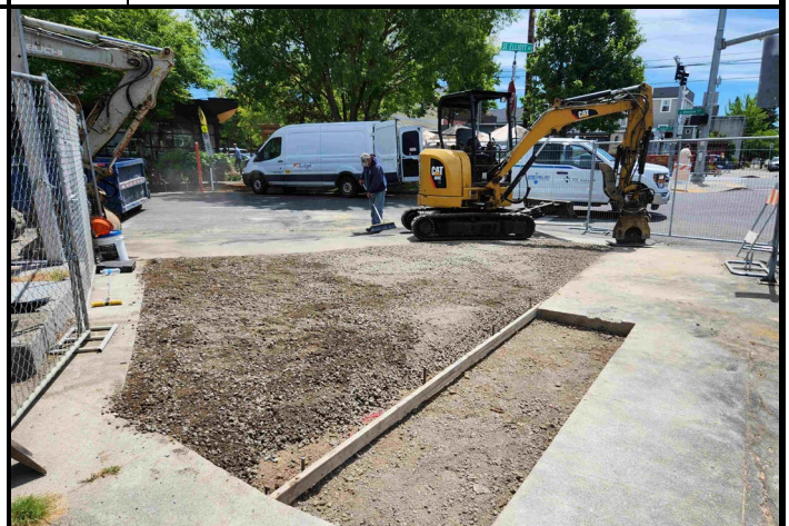
Photo #6: Site Restoration
