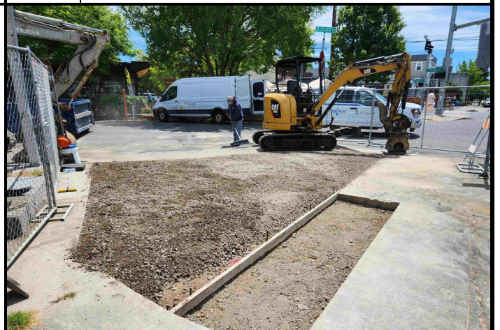
Photo #6: Site Restoration
