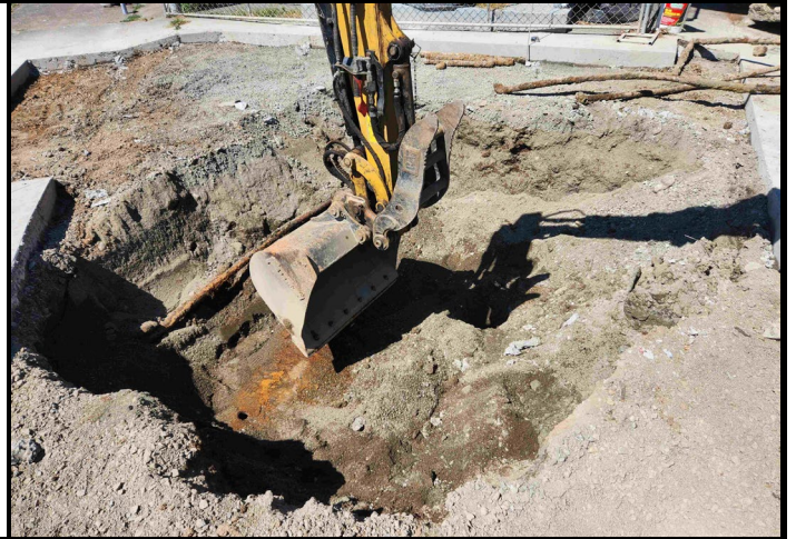
Photo #2: Initial Excavation
