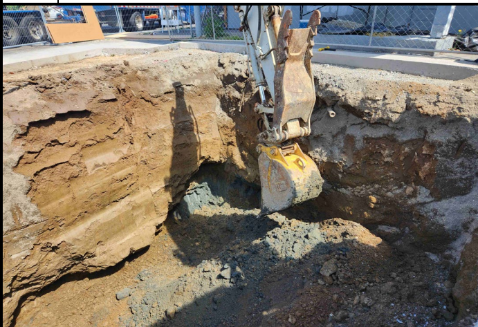
Photo #5: Excavation of PCS
