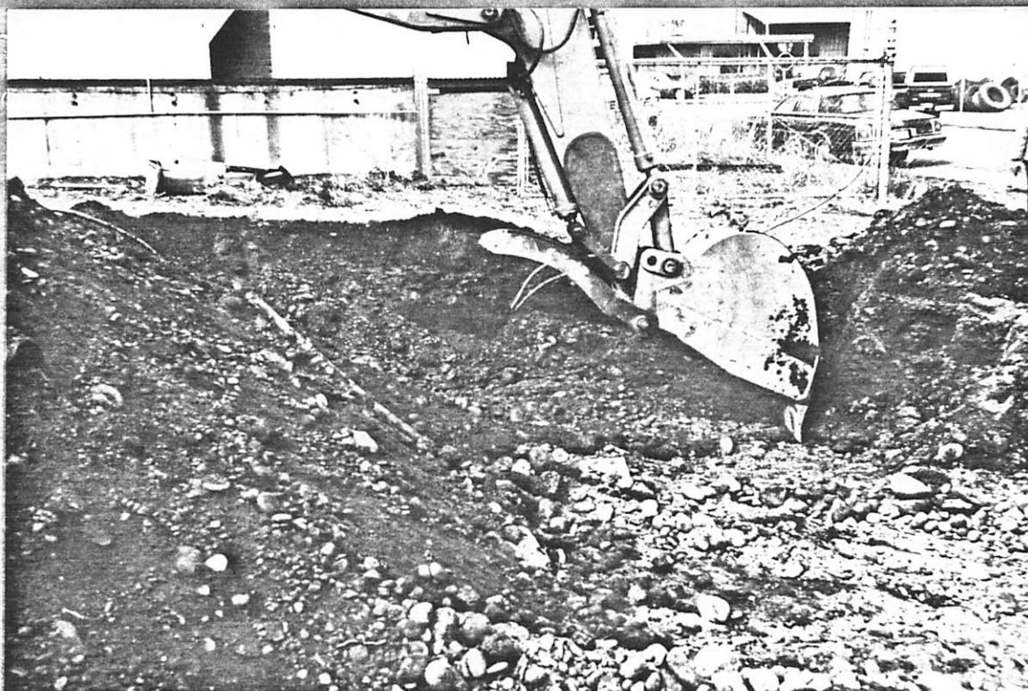
Expansion of the Original UST Excavation Pit to Remove Contamination
