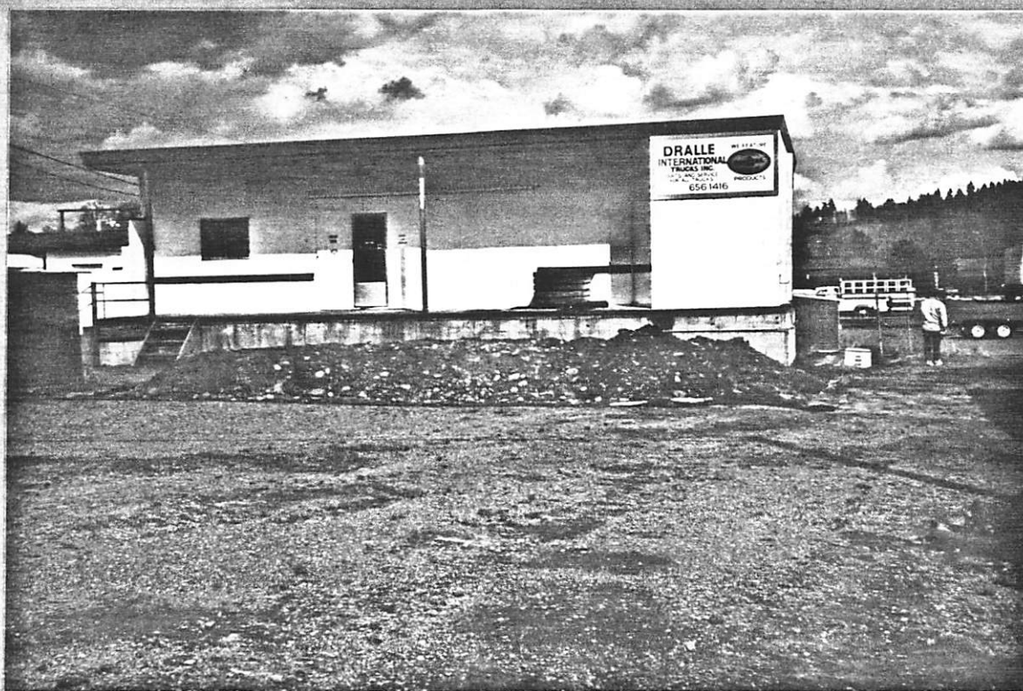
Aeration Stockpile for Gasoline-Contaminated Soil--Early Stages of Construction
