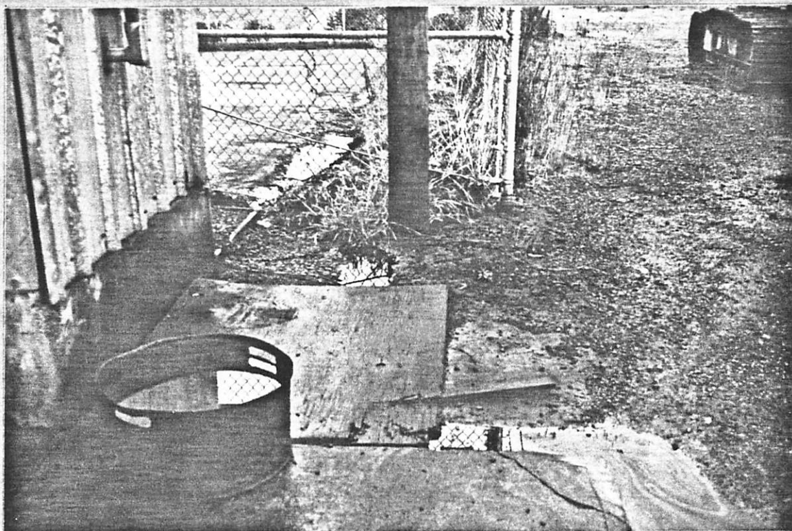
Oil-Contaminated Soil Near the Rear Shop Door Before Excavation
