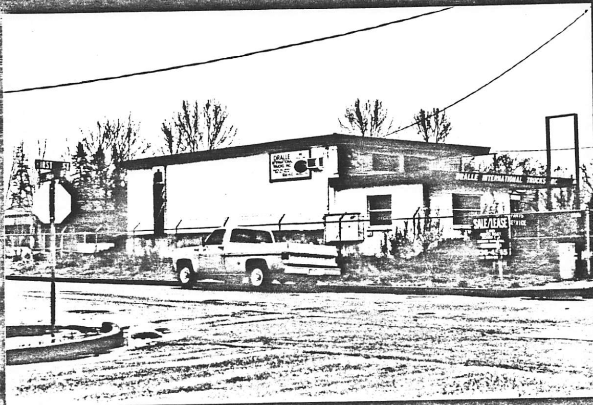
Overview of Property
