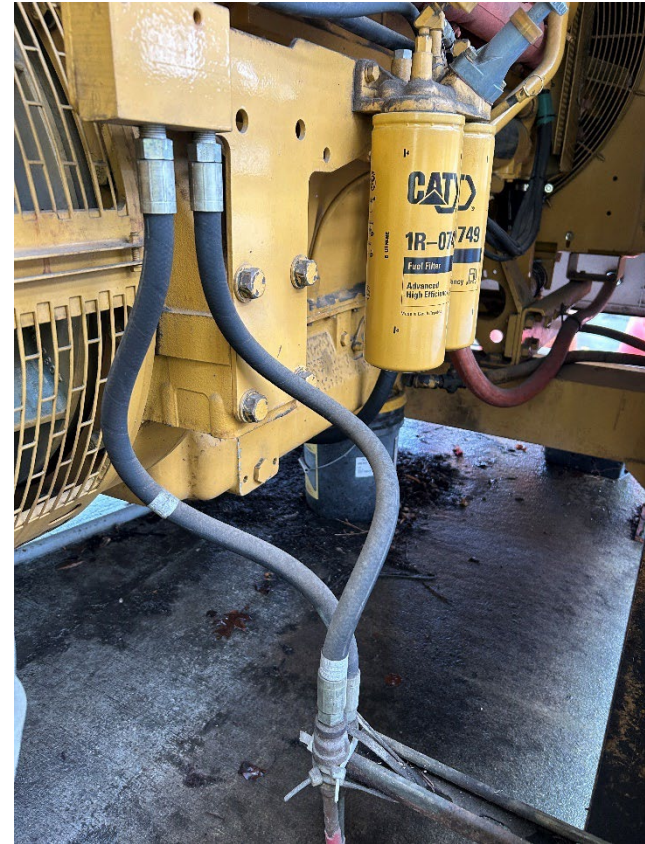
6: Fuel lines into the generator
