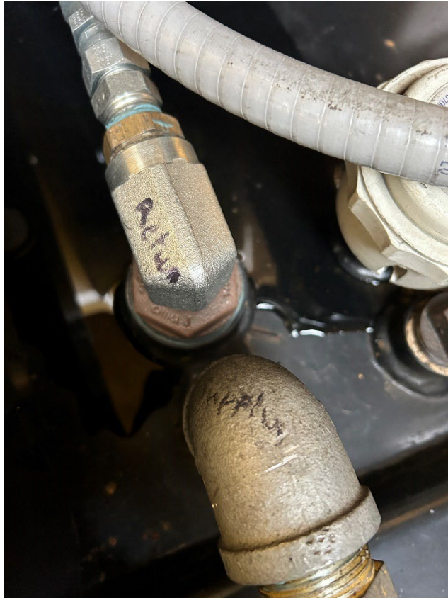
7: Return and supply lines into the generator
