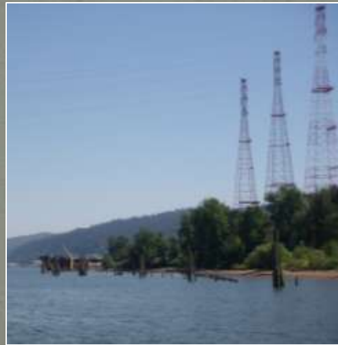
Transmission towers on liquefiable soil
