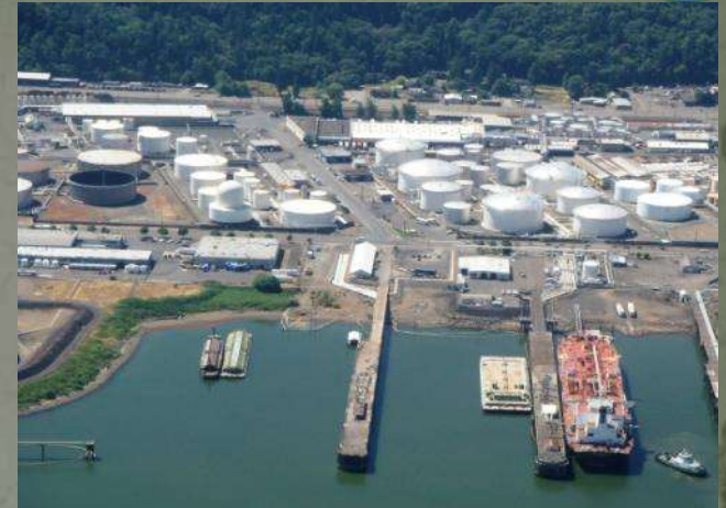
Fuel storage tanks on potentially liquefiable soil in Portland harbor
