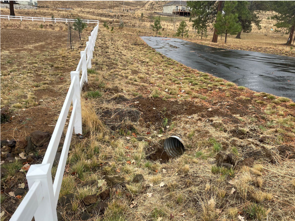
Parcel M – Culvert blockage removed to enable unrestricted capacity.
