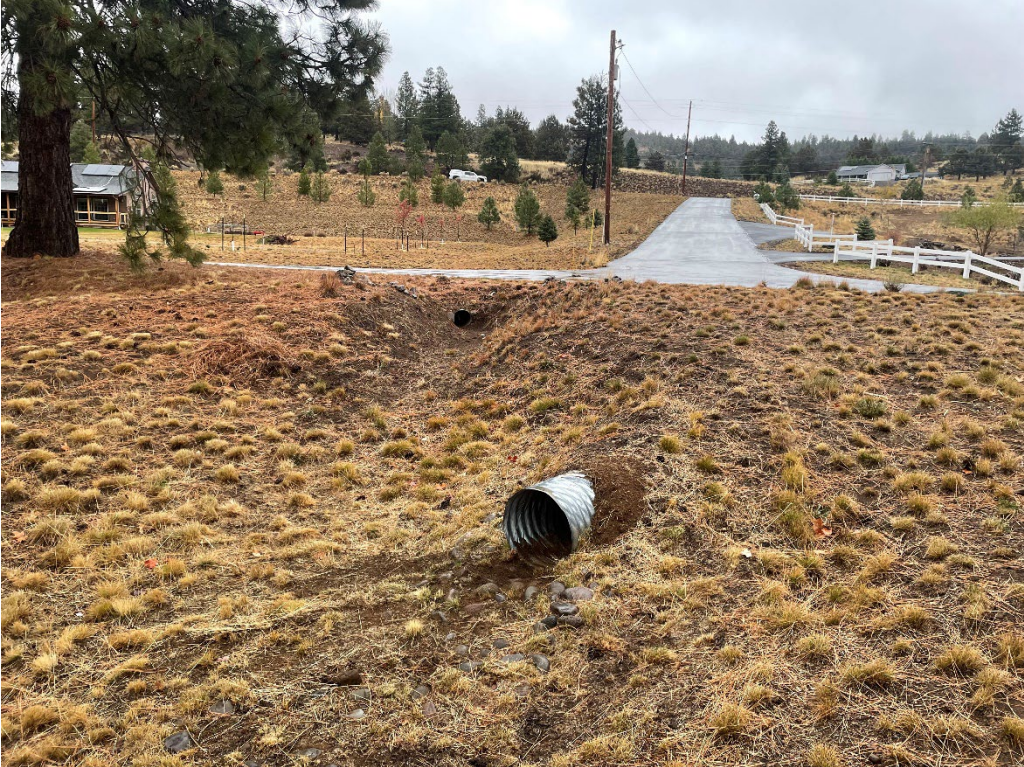
Parcel N – Culvert blockage removed to enable unrestricted capacity.
