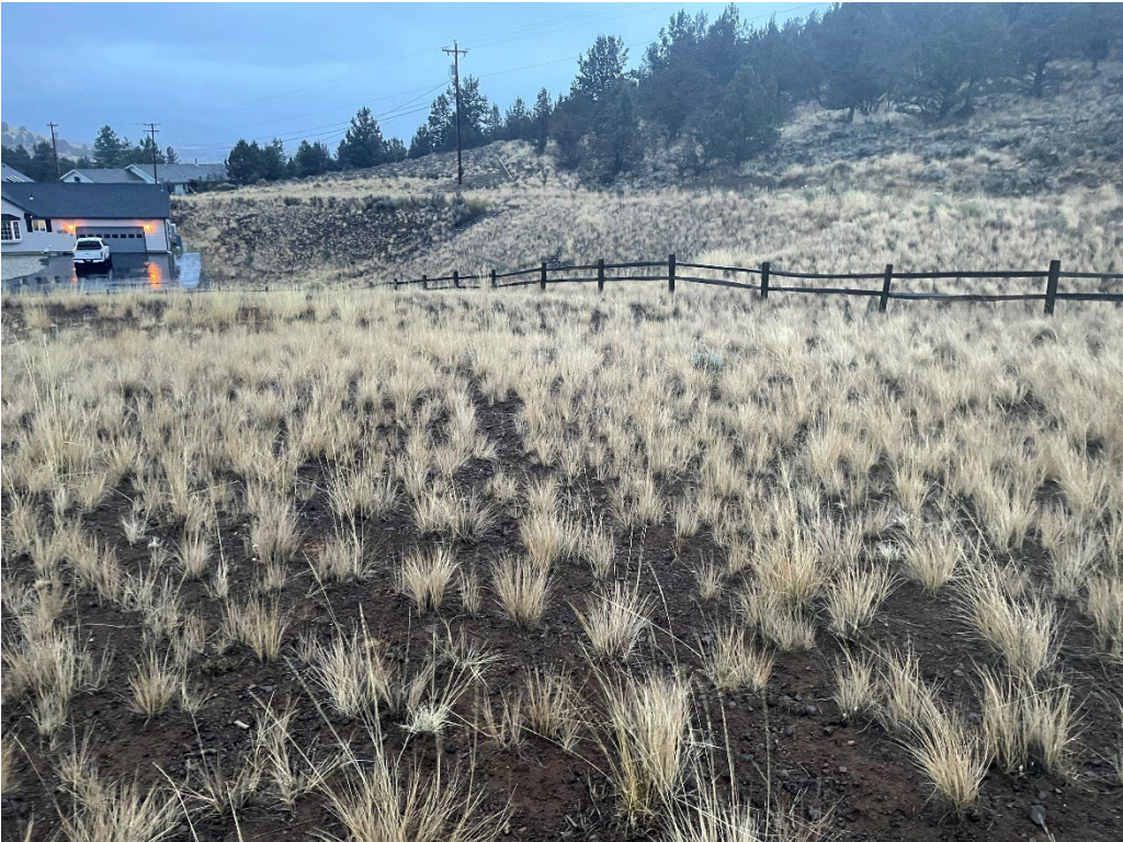
Swimming Pool Repository – No repairs made to gully near south corner of Parcel AG.
