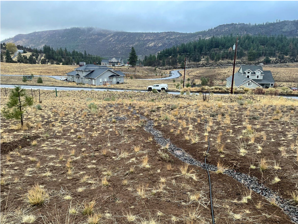
Parcel C – Gullies sufficiently armored with river rock.
