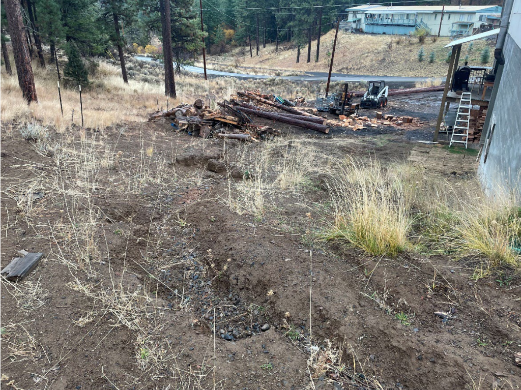
Parcel MBK-G – No repairs made to gully on north side of warehouse.
