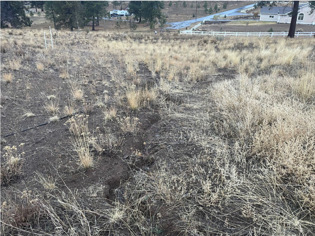
Parcel R – No repairs made to gully near west edge of parcel.
