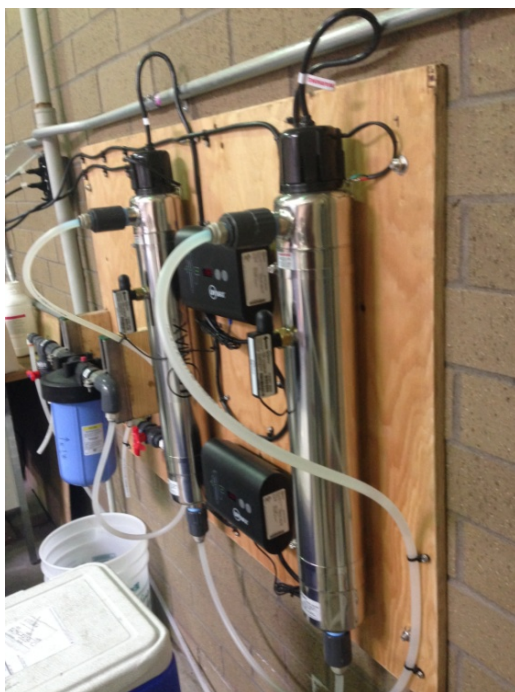
Figure 20 High Dose UV Reactors (two in series) from Trojan Technologies
