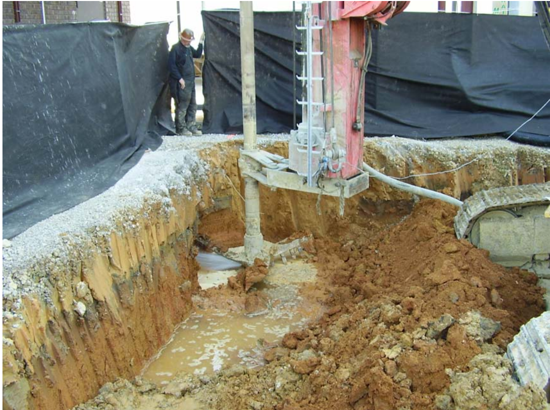
Deep soil mixing rig showing auger head with grout spraying from cutter head.
