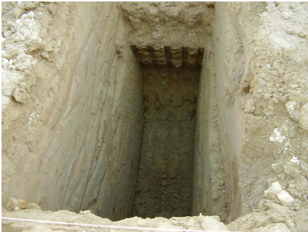
Trench excavated with a track hoe following ISS.
