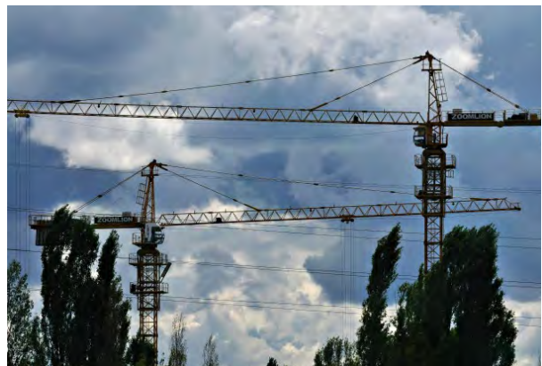
Figure 3: Cranes are especially vulnerable to lightning.
