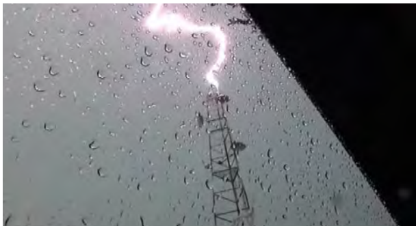
Figure 2: Lightning strikes a communications tower.
