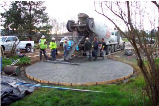
*Using this special type of concrete allows water to seep into the ground rather than running directly to Bear Creek.*
