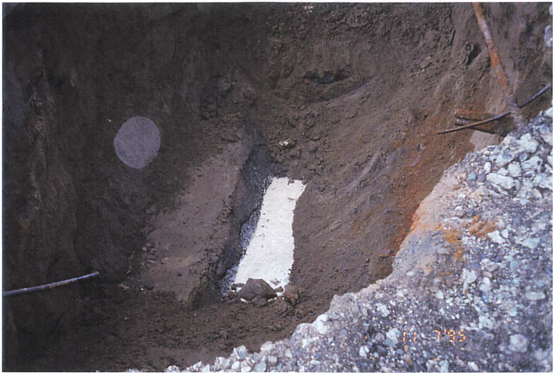
Photograph 7: Bottom of UST excavation immediately after UST removal (Facing southeast)
