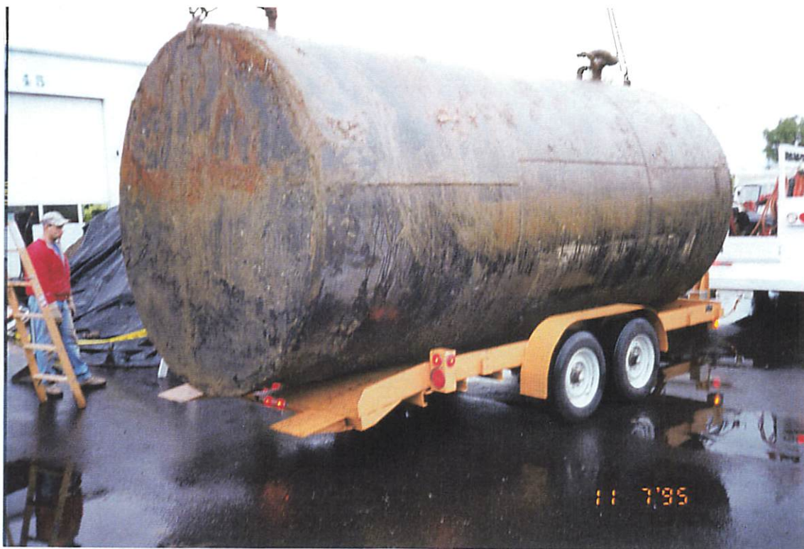
Photograph 4: 6,000-gallon waste oil UST
