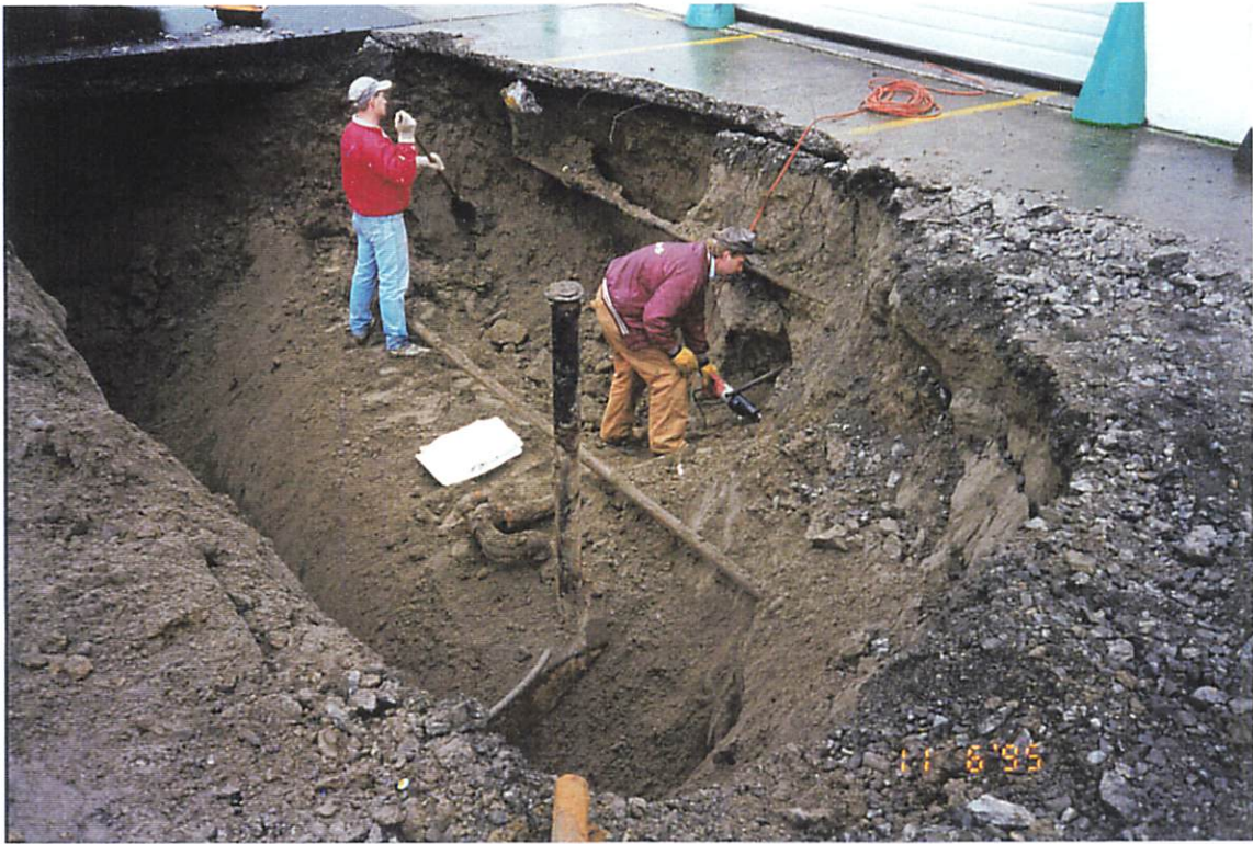
Photograph 1: Uncovering 6,000-gallon waste oil UST (Facing south)
