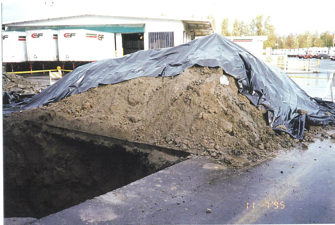
Photograph 9: Excavated soil stockpile (Facing north)
