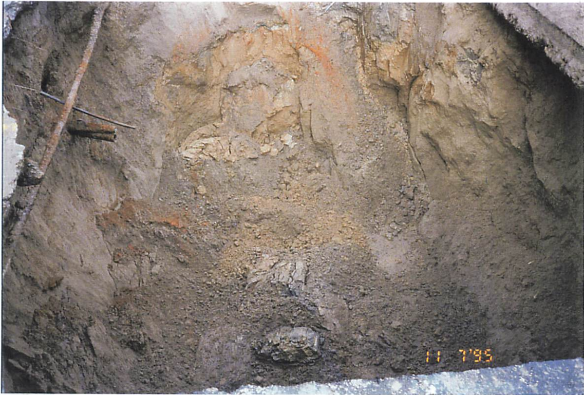
Photograph 8: Bottom of UST excavation after water was soaked up (Facing northwest)
